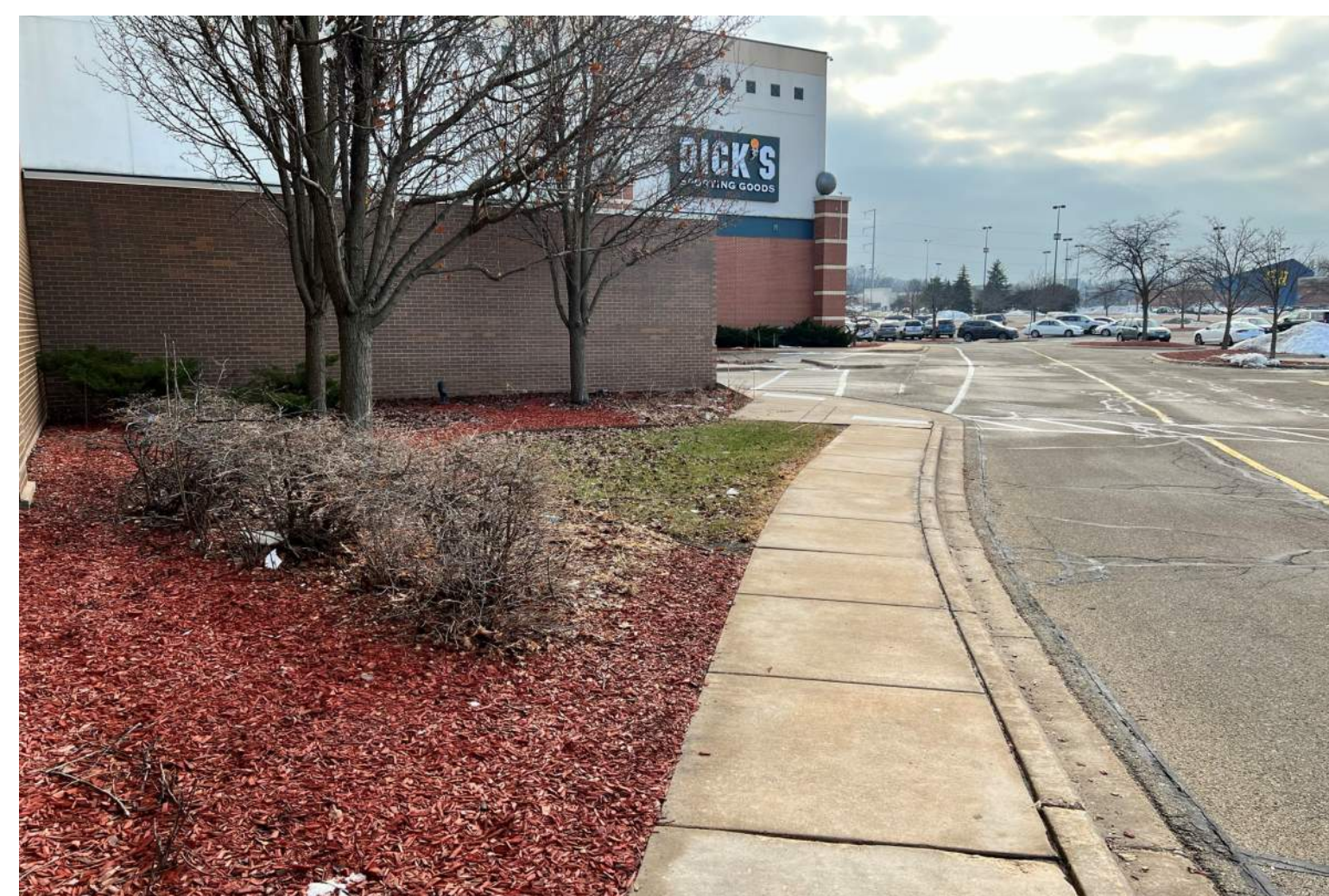
DICK'S SPORTING GOODS NORTH EXTERIOR WALL
