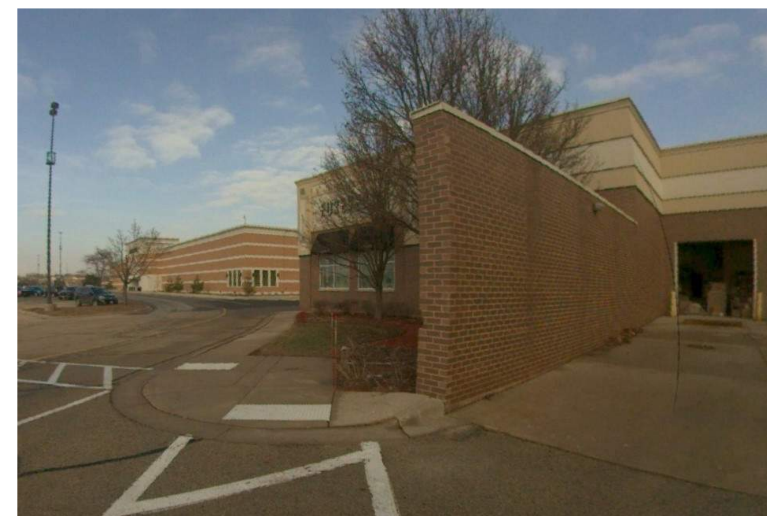
PLANET FITNESS WEST EXTERIOR WALL LOOKING TOWARD VON MAUR
