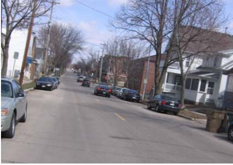
Mifflin and Franklin, looking northwest (good condition)
