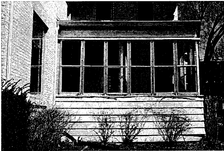
View of original porch columns, relocated to side porch.
