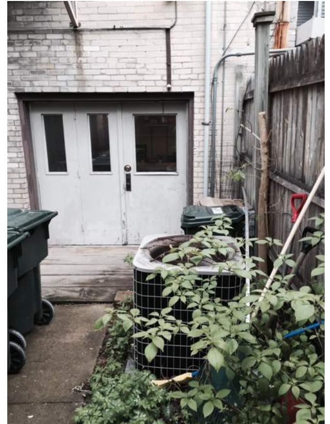
Rear of 409 E. Main Street
