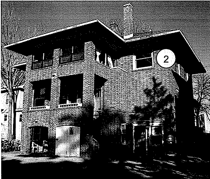
Southeast Elevation (Back)
