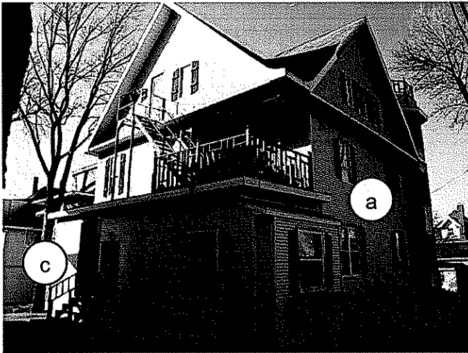
Northeast and Northwest Elevations (Back)
