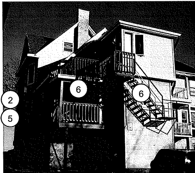
Southeast Elevation (Back)
