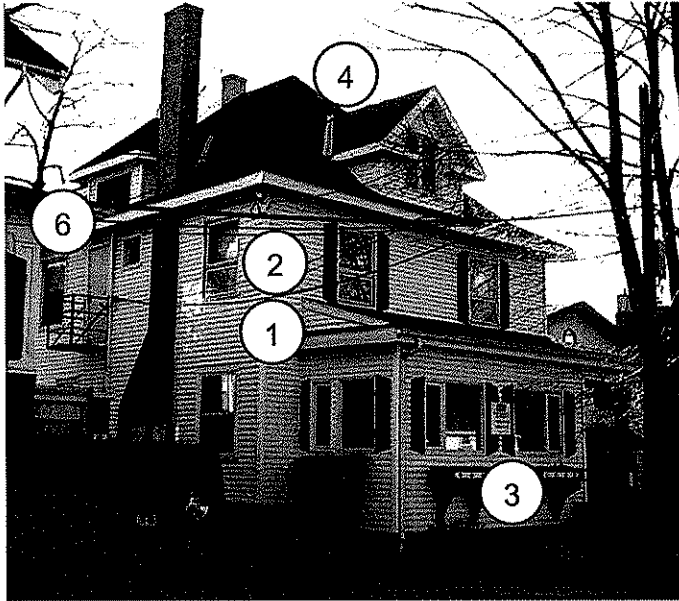
Southwest Elevation (Front)
