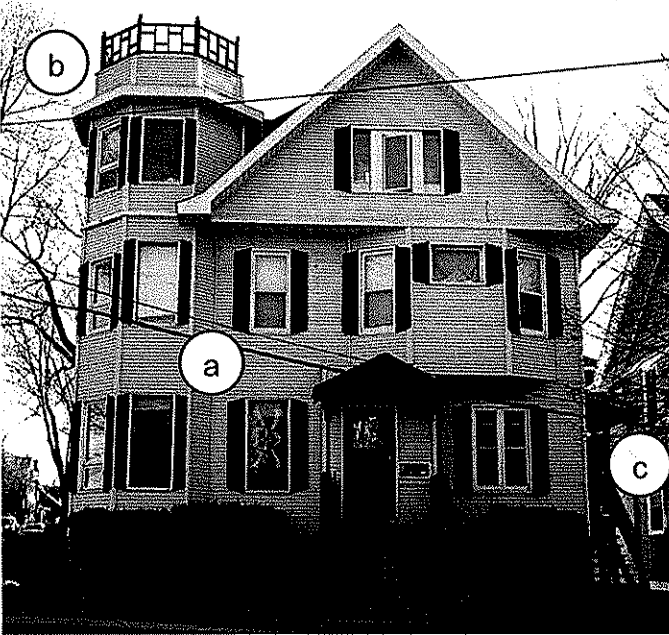
Southwest Elevation (Front)
