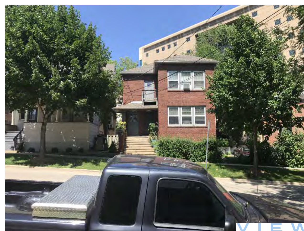
VIEW EAST SIDE OF HENRY STREET
