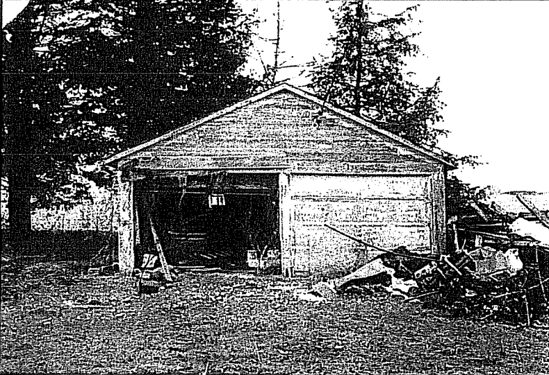
East Side of Garage Looking West
