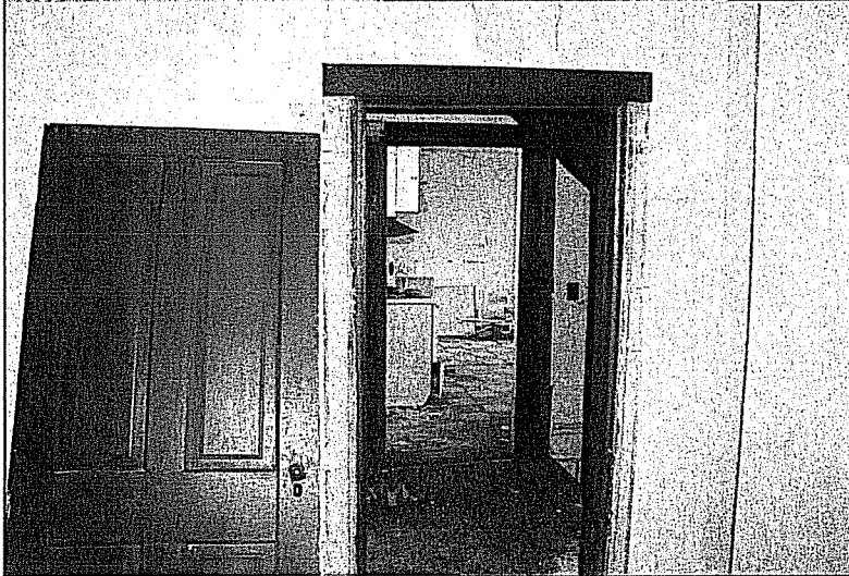
Looking into Kitchen From Bedroom
