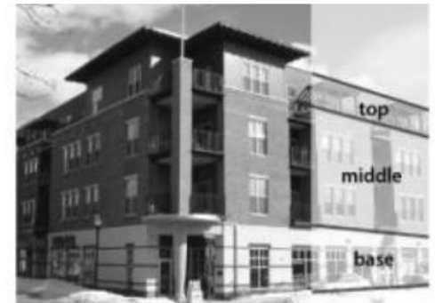
Figure D6 Building Articulation
