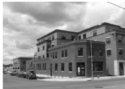
Figure D3 Variation in Roof Lines
