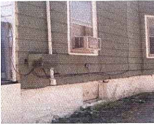
The exterior foundation of 419/421 contains painted concrete block.
