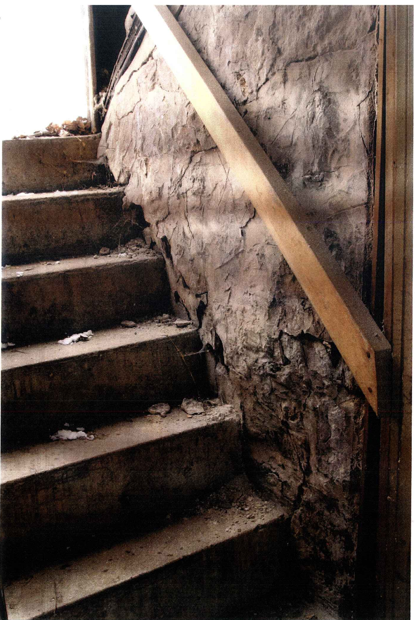
415 W. DAYTON – BASEMENT WALL. NOTE: SLOPING, CRUMBLING, PUSHED-IN WALL
