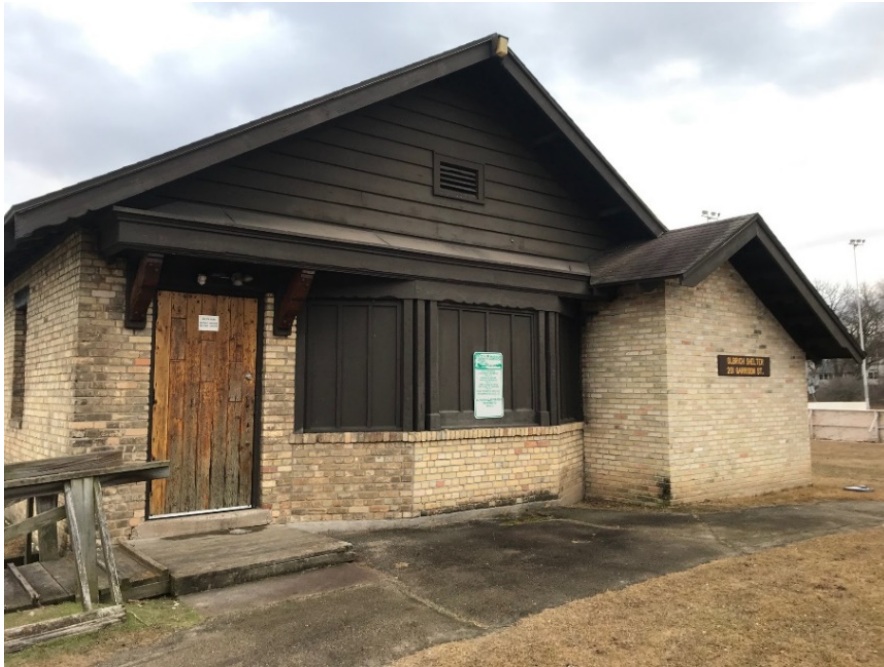
OLBRICH SHELTER ROOF REPLACEMENT
