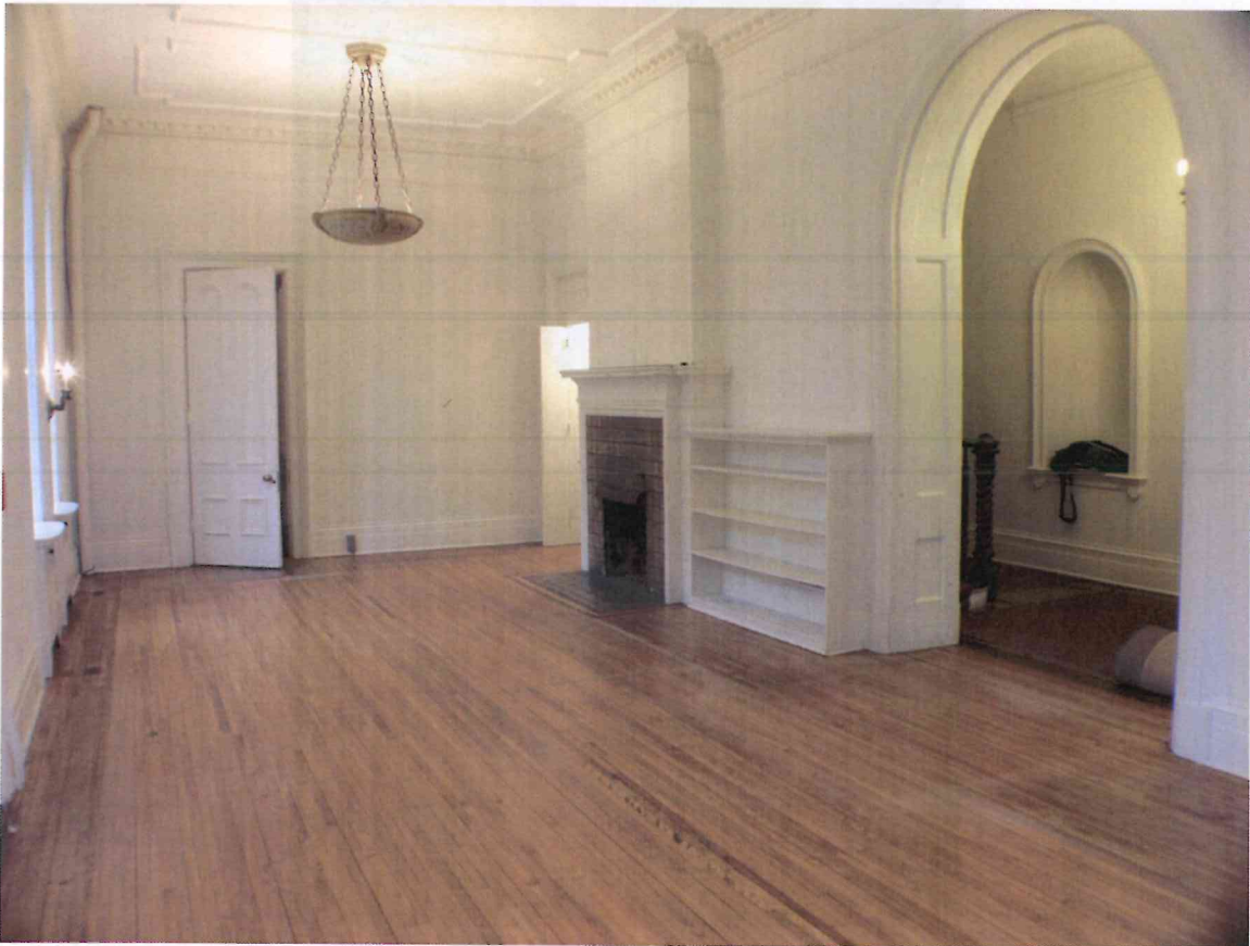
Interior, main dining room
