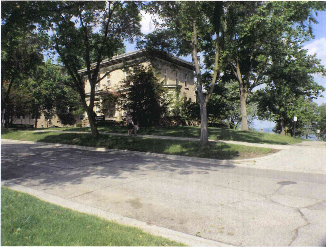
Front elevation from north
