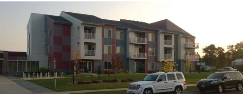
VIEW OF BUILDING A, 10202 RUSTLING BIRCH RD.
