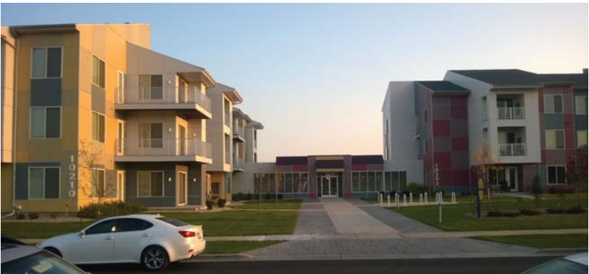
VIEW OF 10202, 10206, 10210 RUSTLING BIRCH RD.
