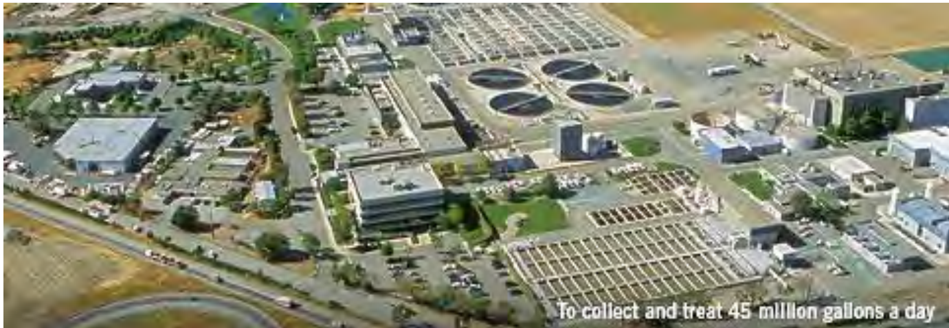
Central San System Site
