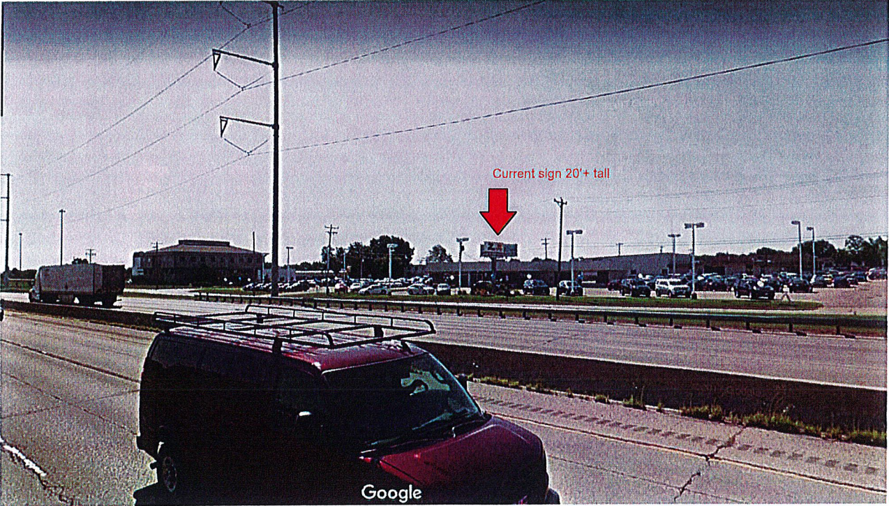
View looking southeast toward dealership from hwy
