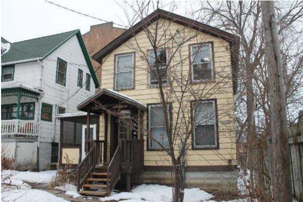
Photo 296: 410 1/2 East Washington Avenue, Exterior, facing northwest
