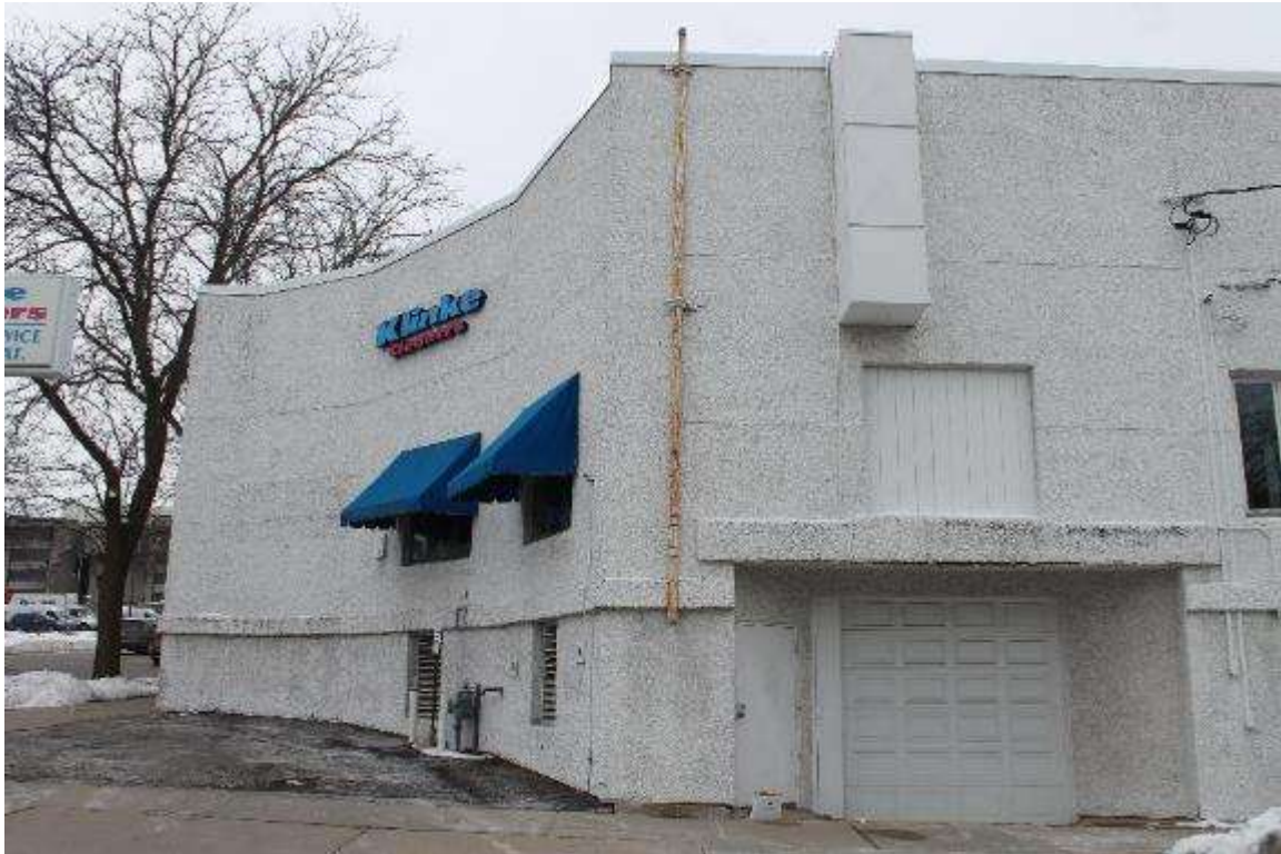
Photo 328: 412-414 East Washington Avenue, Exterior, facing southwest
