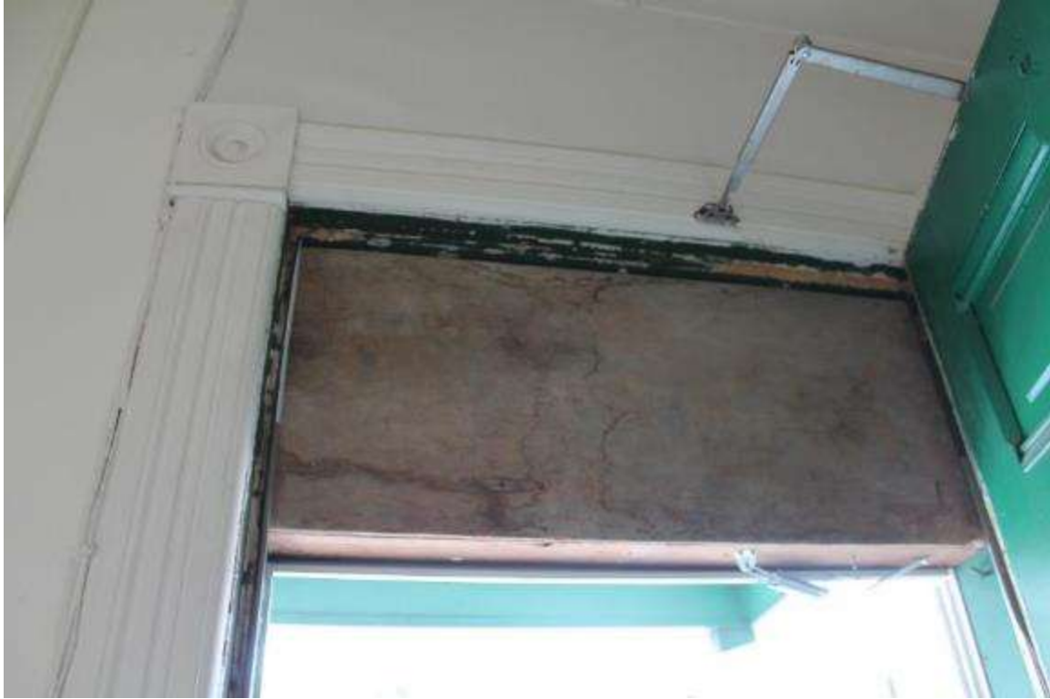
Photo 13: 9 North Hancock Street, Interior, first floor entryway
