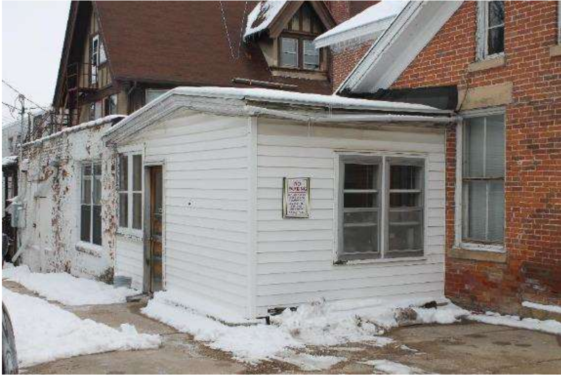
Photo 147: 402-408 East Washington Avenue, Exterior, facing east
