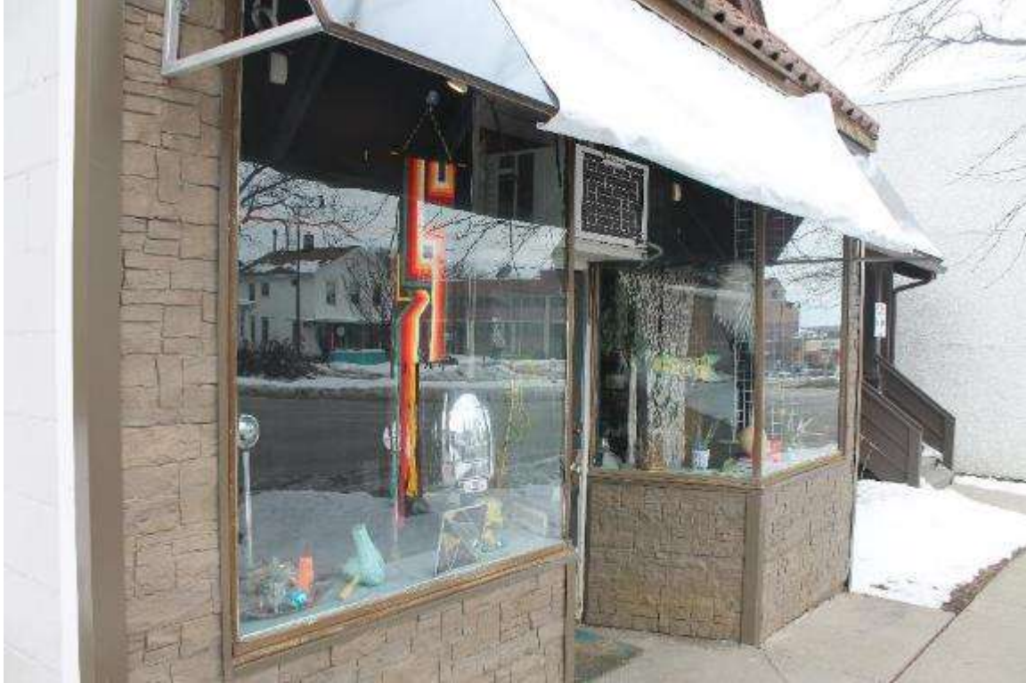
Photo 161: 402-408 East Washington Avenue, Exterior, facing north
