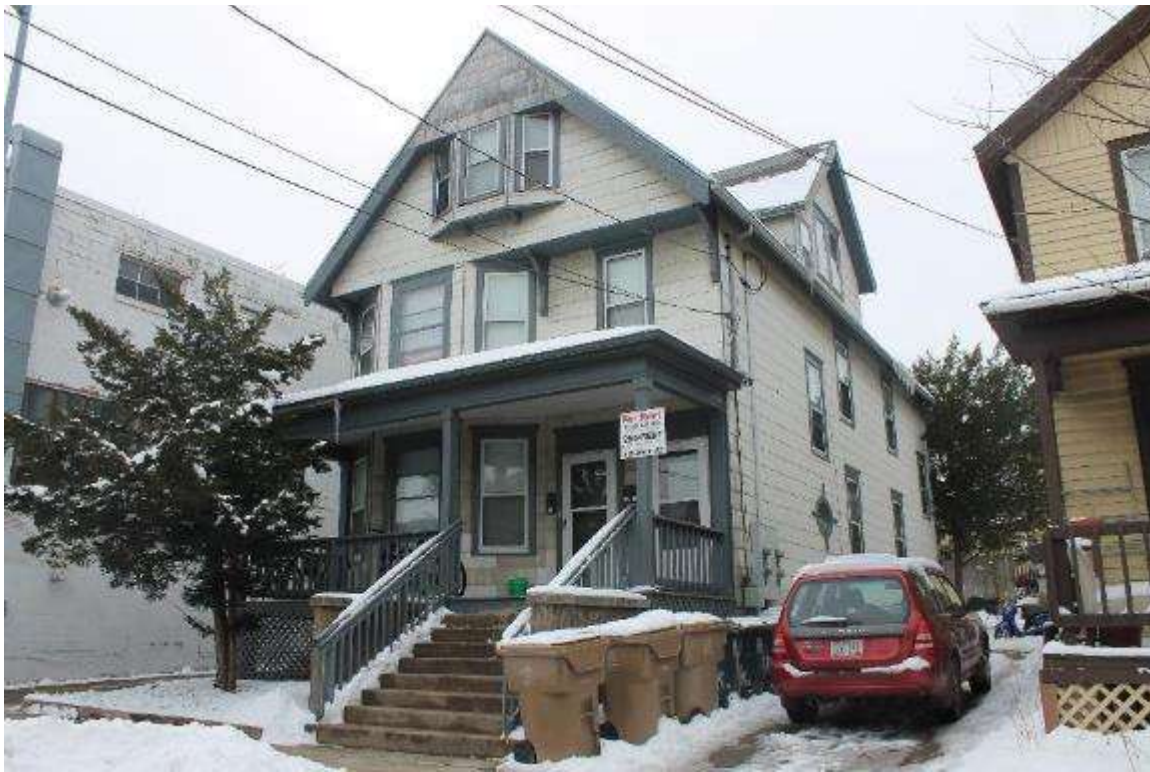
Photo 51: 8-10 North Franklin Street, Exterior, facing south
