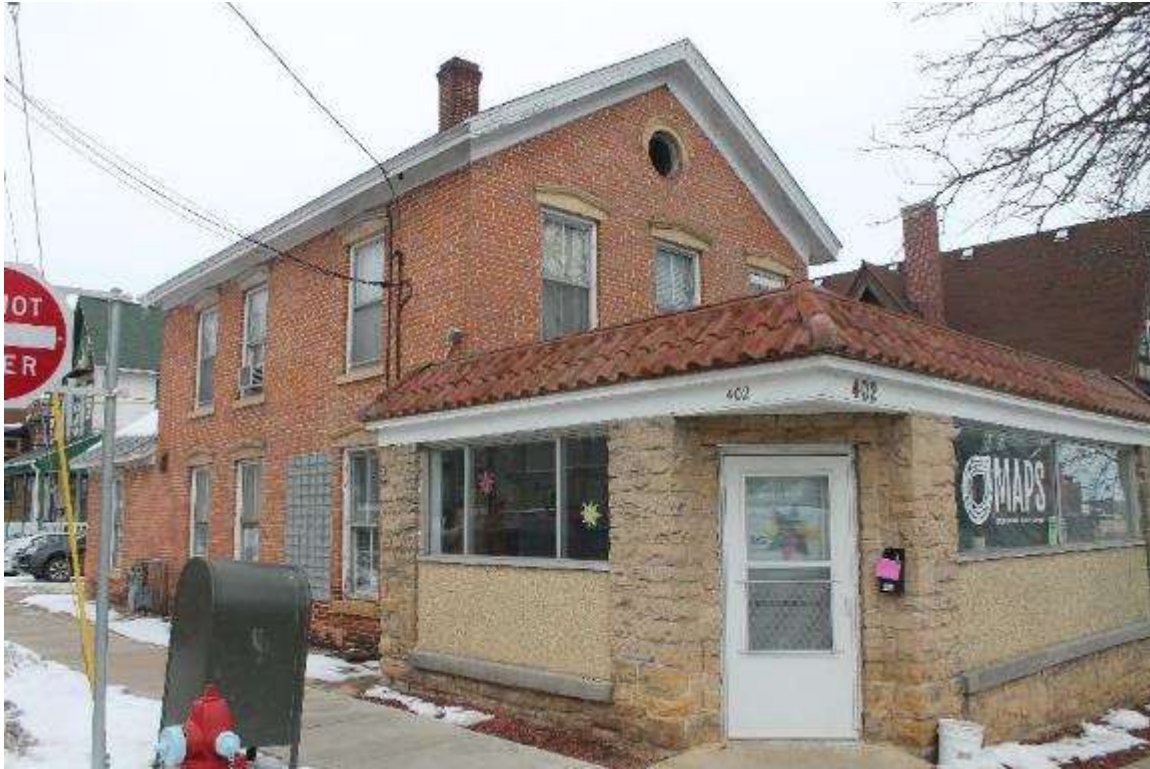
Photo 135: 402-408 East Washington Avenue, Exterior, facing north
