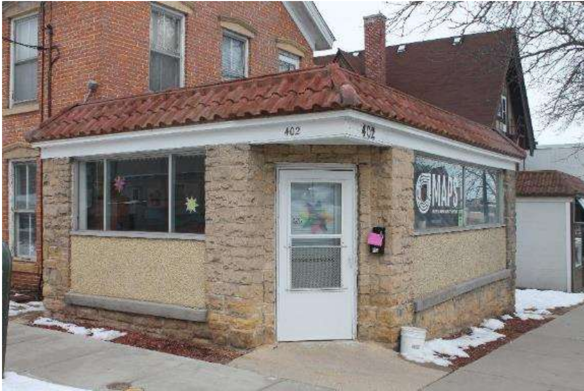
Photo 136: 402-408 East Washington Avenue, Exterior, facing north
