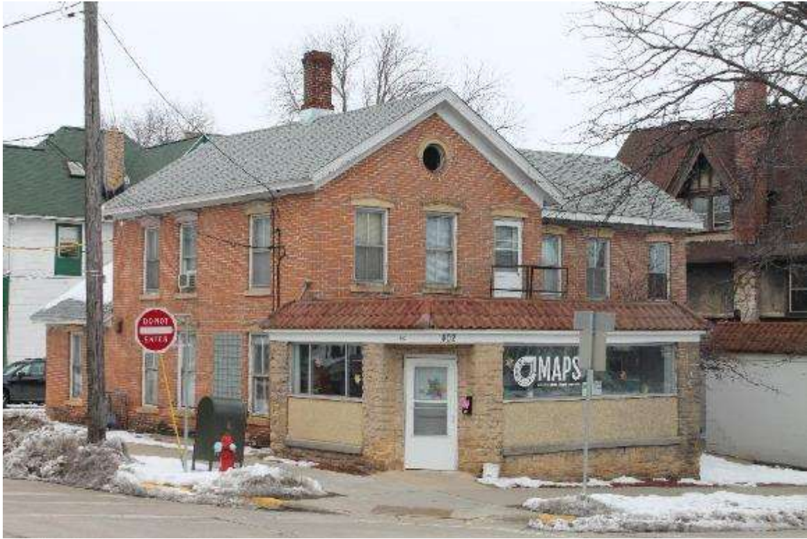
Photo 132: 402-408 East Washington Avenue, Exterior, facing north
