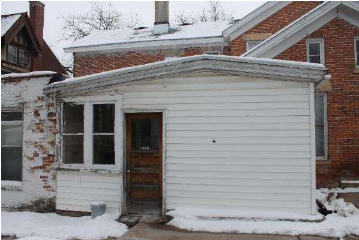
Photo 148: 402-408 East Washington Avenue, Exterior, facing southeast
