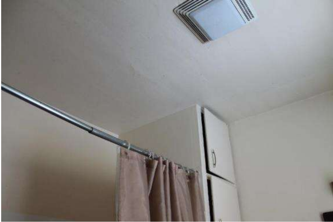
Photo 215: 402-408 East Washington Avenue, Interior, second floor unit 4
