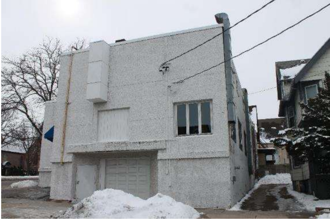
Photo 329: 412-414 East Washington Avenue, Exterior, facing southwest
