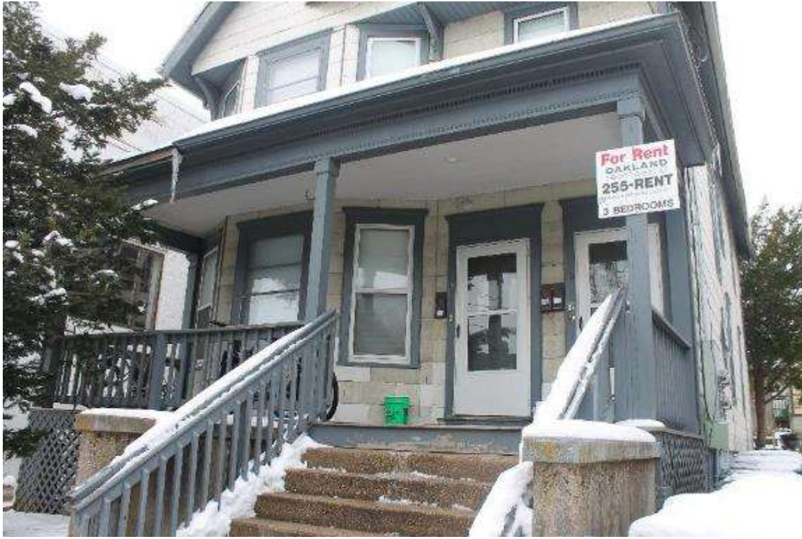
Photo 52: 8-10 North Franklin Street, Exterior, facing south
