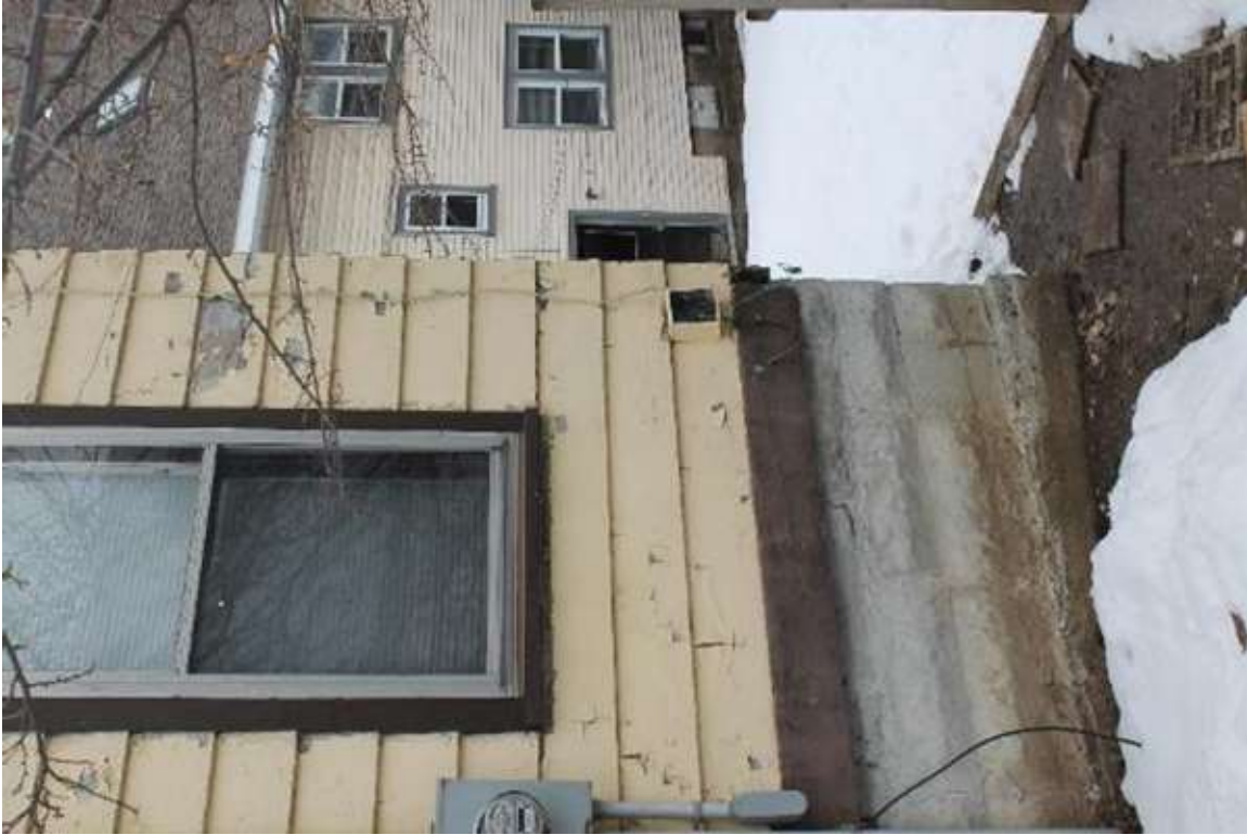
Photo 298: 410 1/2 East Washington Avenue, Exterior, facing north
