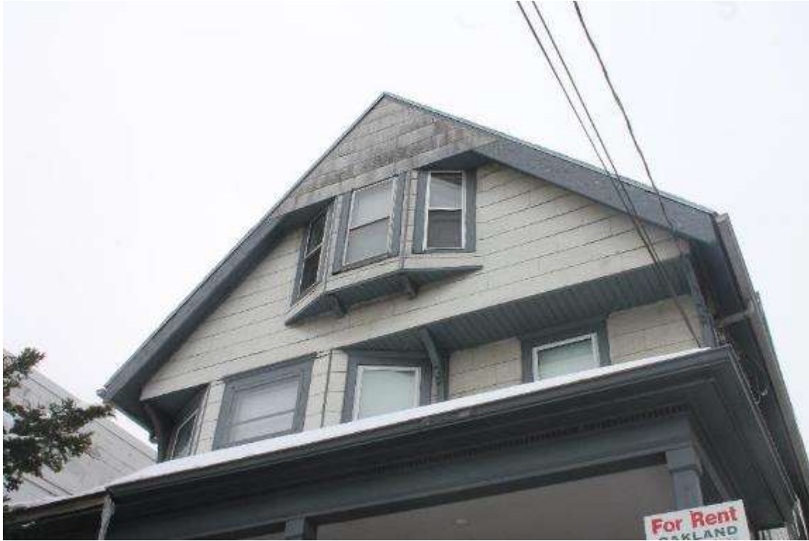
Photo 53: 8-10 North Franklin Street, Exterior, facing south
