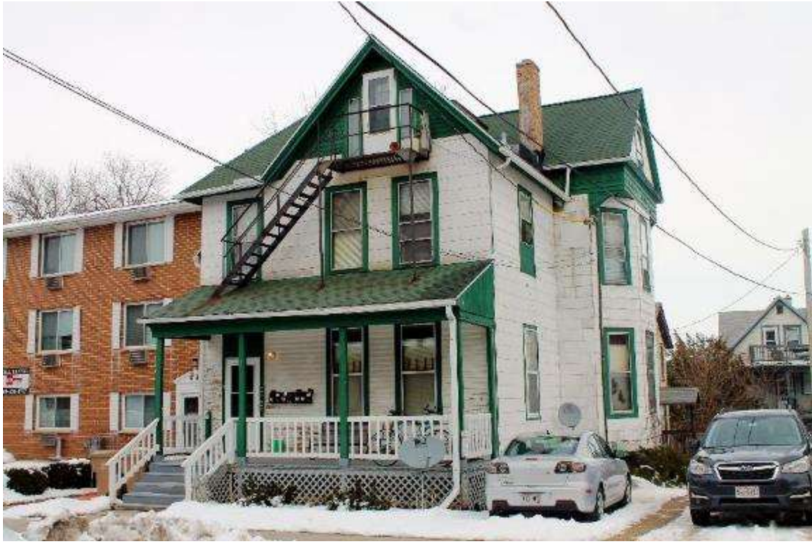
Photo 1: 9 North Hancock Street, Exterior, facing northeast
