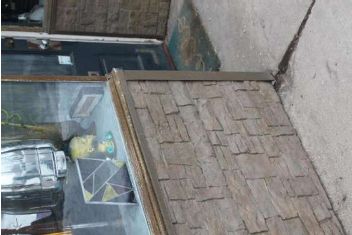
Photo 163: 402-408 East Washington Avenue, Exterior, facing north
