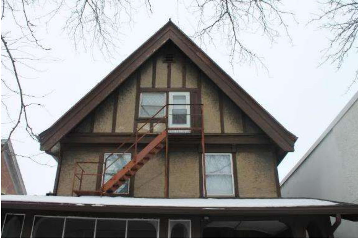
Photo 229: 410 East Washington Avenue, Exterior, facing northwest
