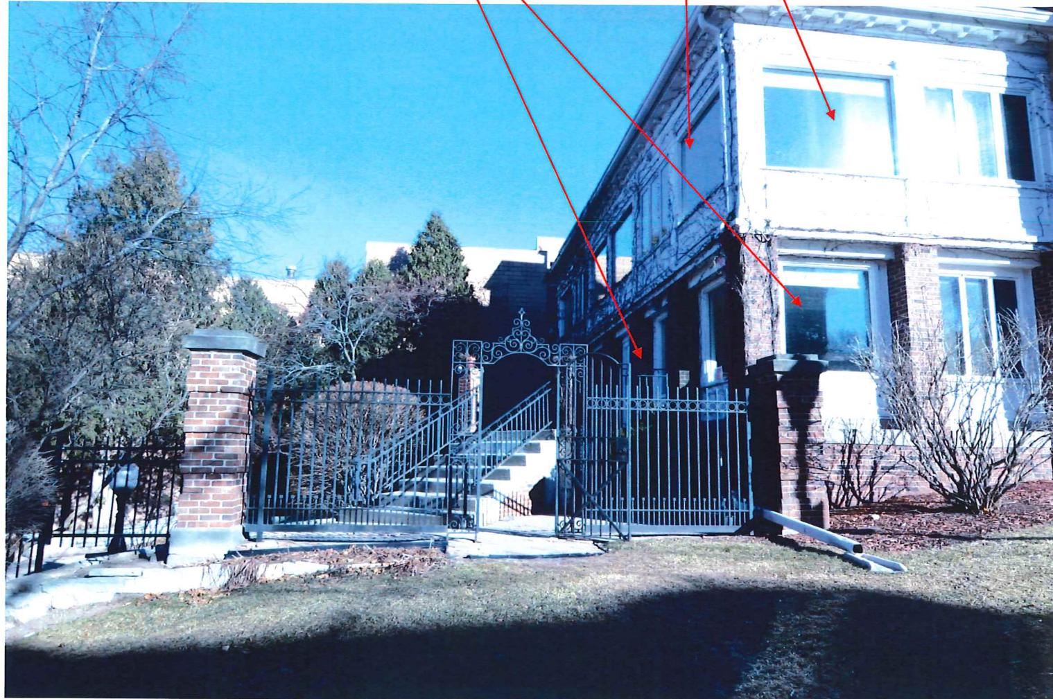
Rear/Side Elevations (from southwest) PHOTO 3
