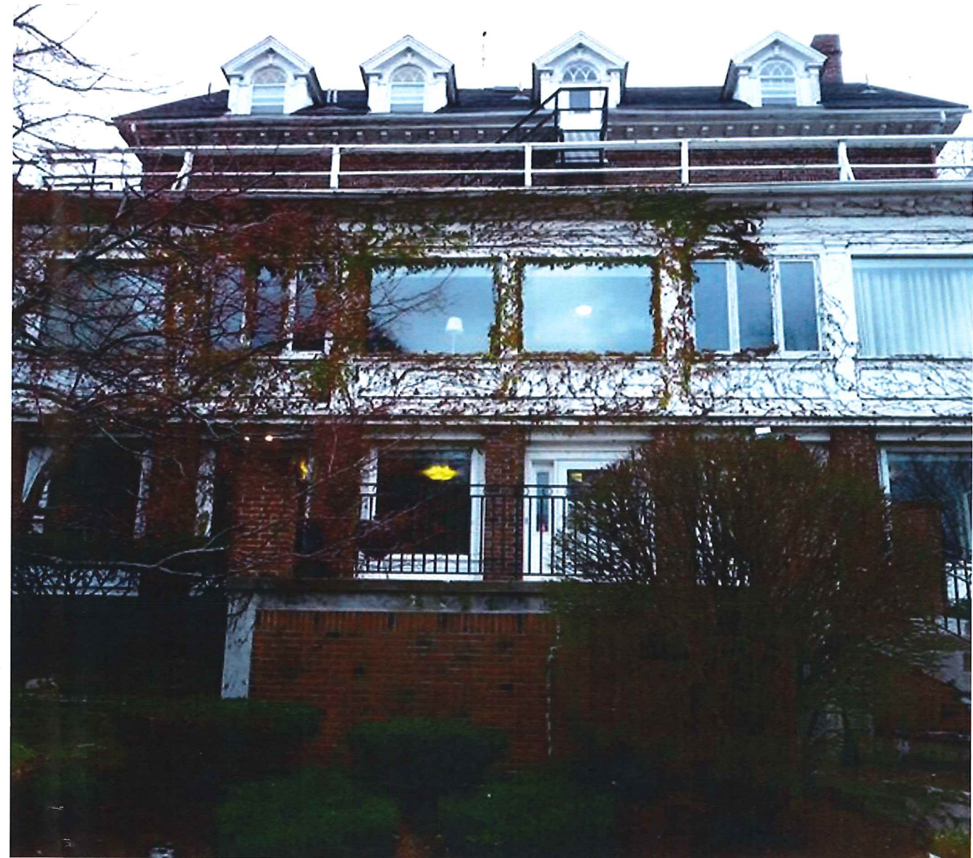
Rear Elevation (from west) PHOTO 2
