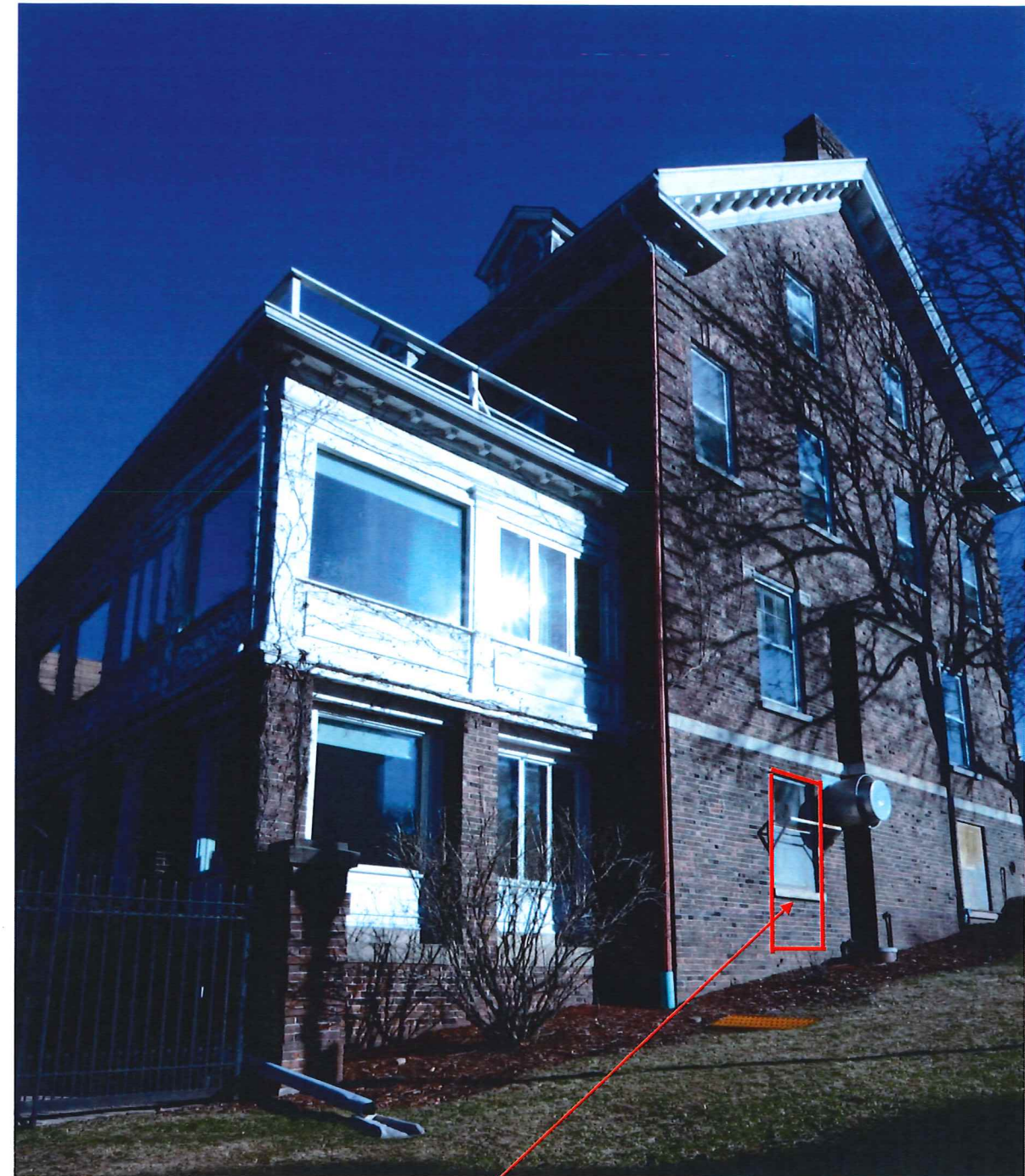
New door (#B-201-1) in Kitchen to replace non-original infill panel
