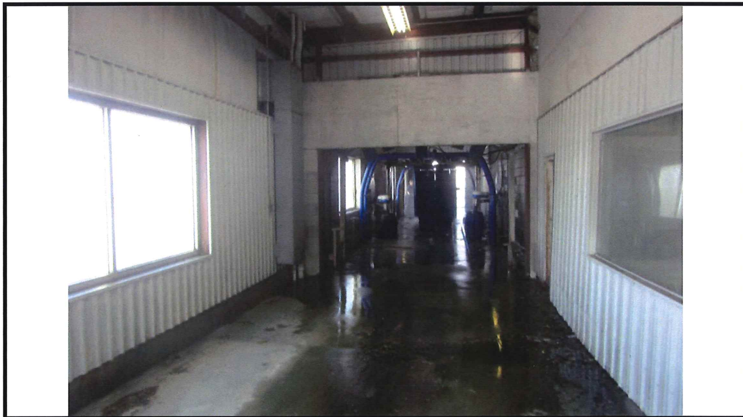
06 - INSIDE OF CAR WASH AREA
