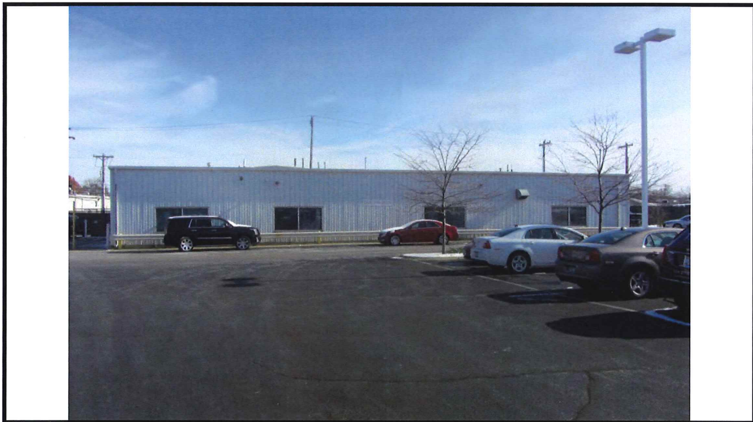
02 – WEST SIDE OF EXISTING BUILDING
