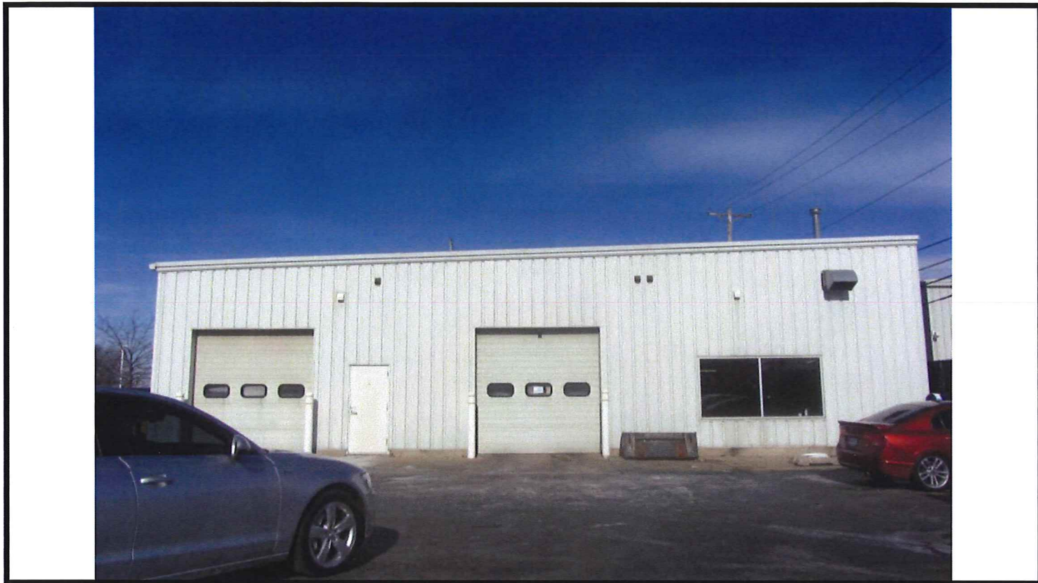
01 – SOUTH SIDE OF EXISTING BUILDING
