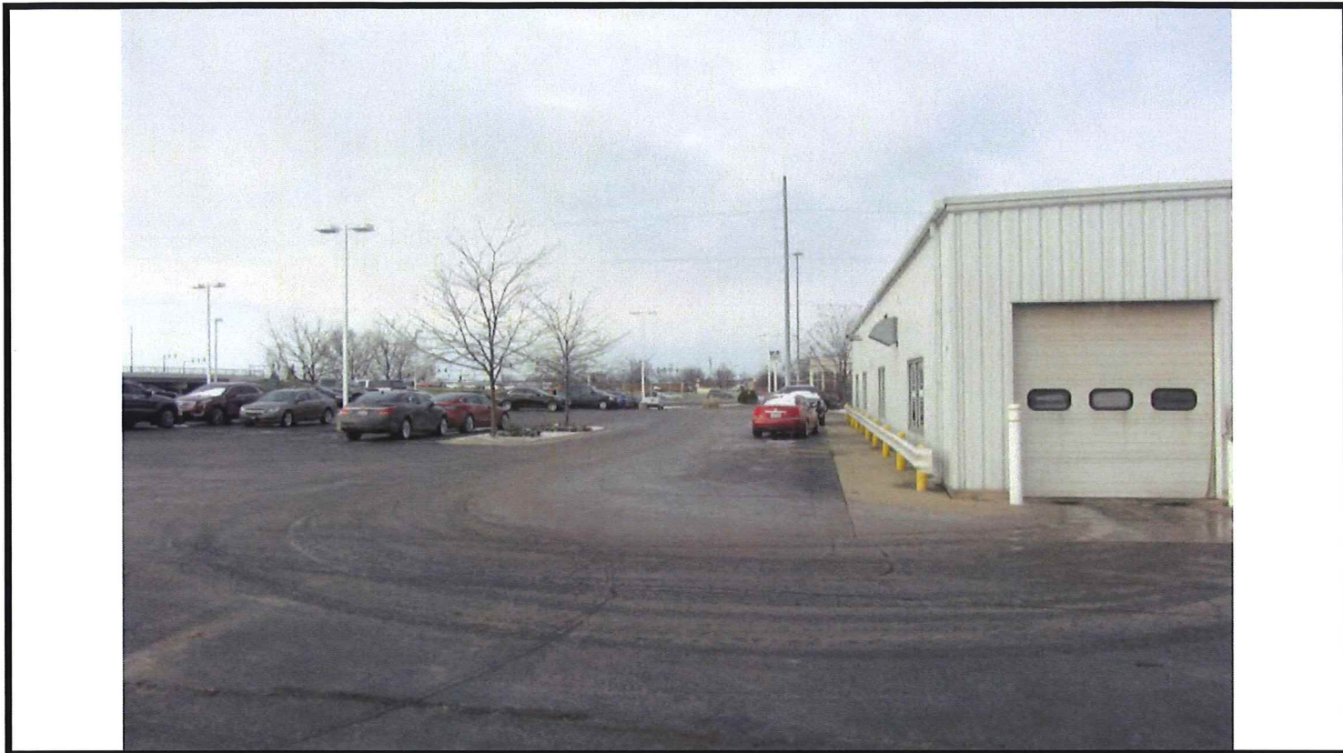
05 - LOOKING NORTH ALONG WEST SIDE OF EXISTING BUILDING
