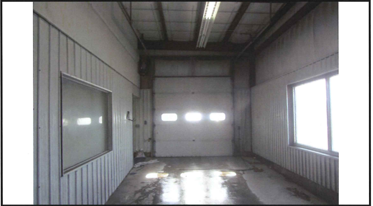
07 - INSIDE OF CAR WASH AREA
