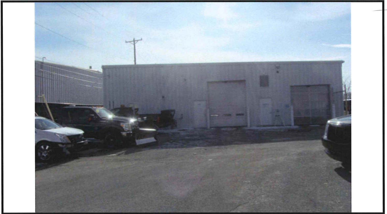
03 – NORTH SIDE OF EXISTING BUILDING
