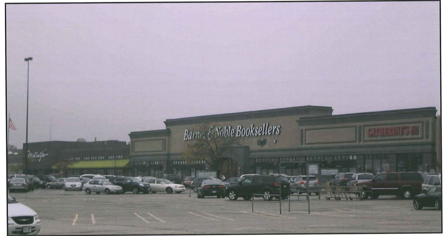
Adjacent Property to Southwest
