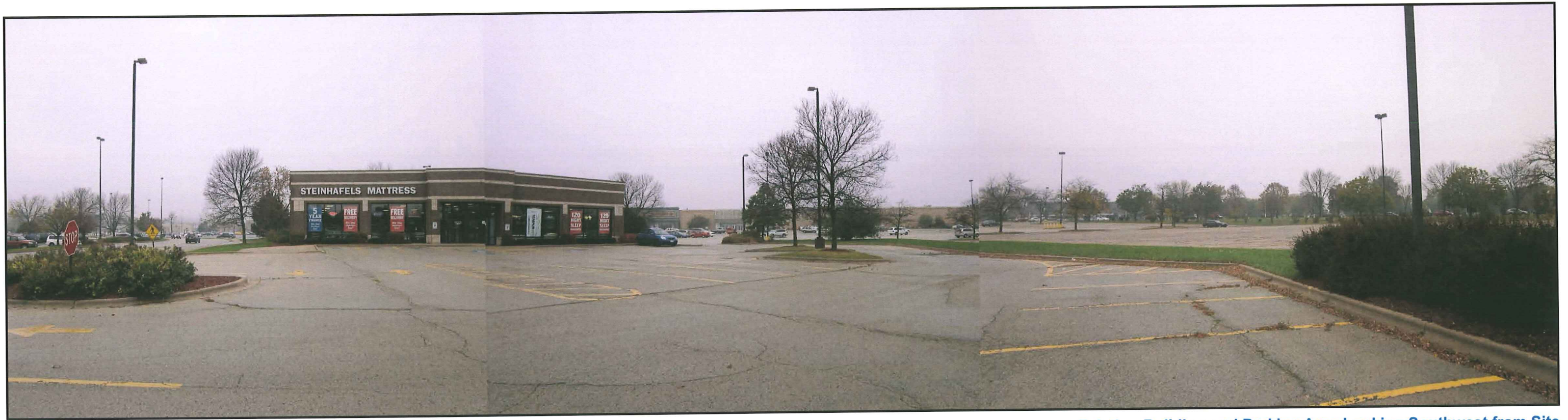
Existing Building and Parking Area Looking Southwest from Site
