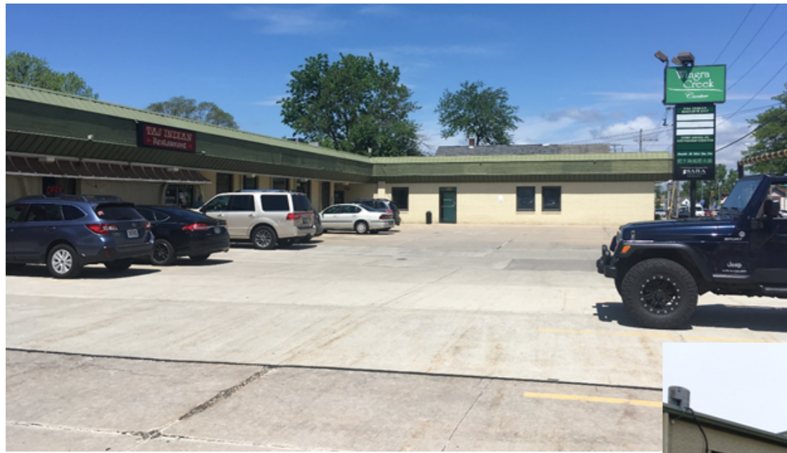
Exterior from Southeast
