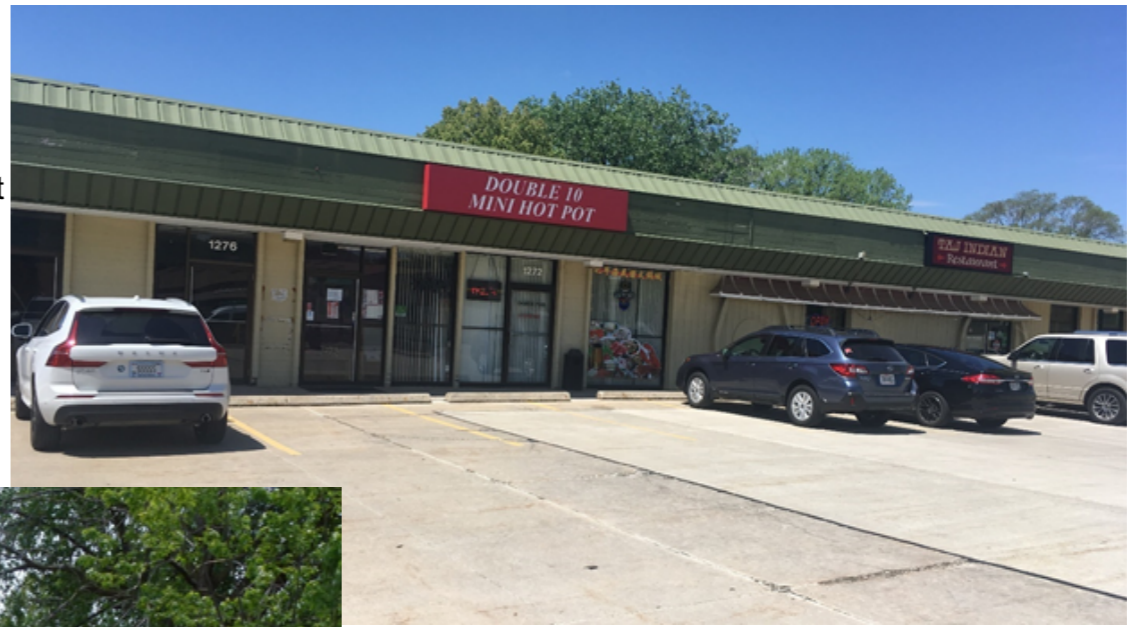
Exterior looking West
