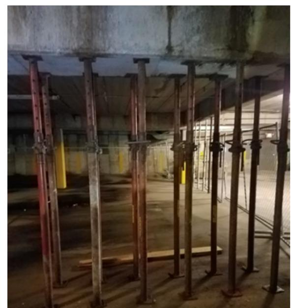
Interior lower level parking area, showing fenced-off area with temporary shoring posts
