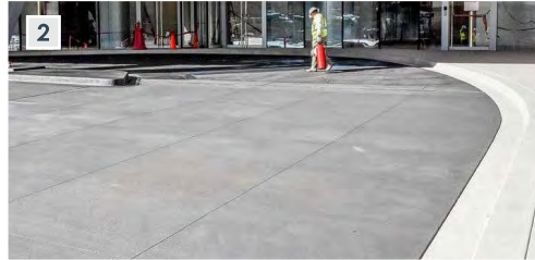
CONCRETE - BROOM FINISH
