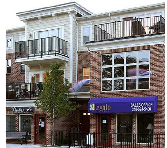
Three-story building with residential units above retail uses
