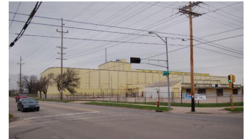
Fertilizer Plant- Main Granulation Building
