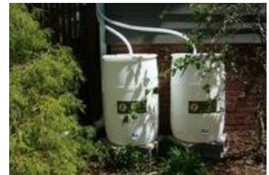
Cisterns and small rain barrels like these may be incorporated for rainwater collection and reuse.
