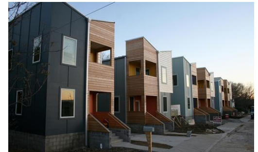
Unique multifamily residential development with a passive solar design
