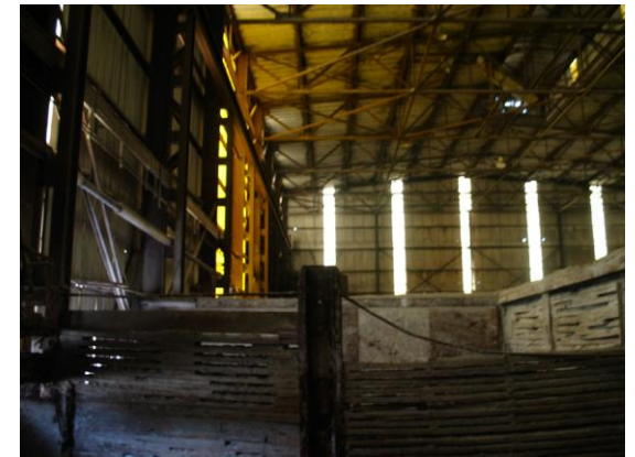
Interior of the main granulation building
