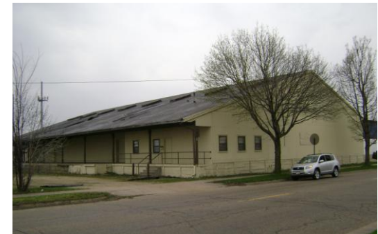
Vacant warehouse in the Commercial Triangle
