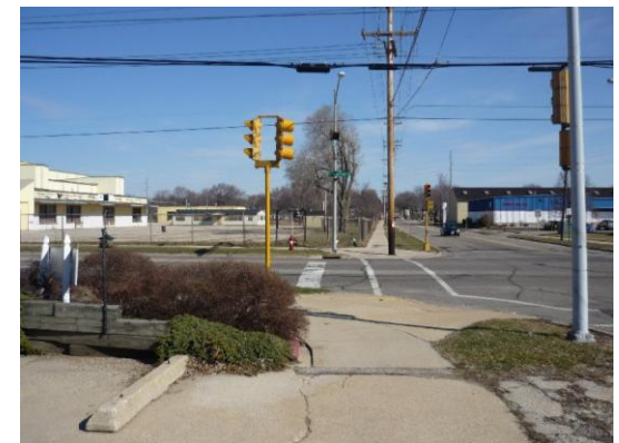
Sidewalks at the existing intersection of Dempsey and Cottage Grove Rd, with diagonal ramps leading into the intersection or obstructed by poles
