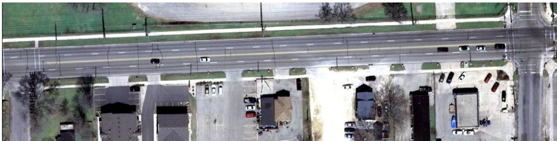
Aerial photo of Cottage Grove Road illustrating the number of driveways servicing individual parcels
