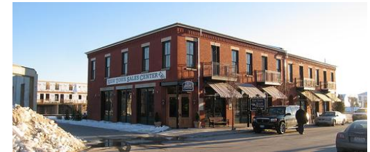
Two-story building with residential units above retail uses
