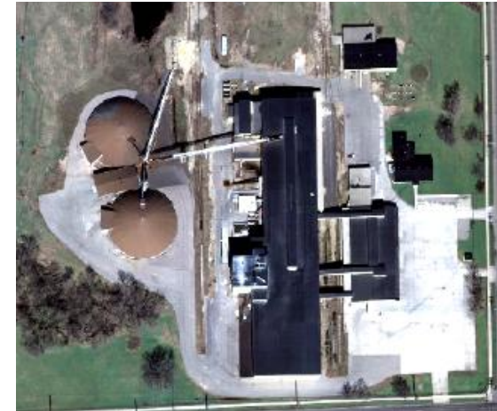
Aerial view of the former Royster-Clark fertilizer plant
