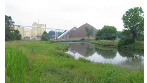
Fertilizer Plant- Storage Domes and Ponds
