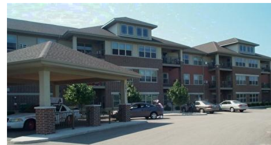
Buildings similar to this senior housing development may be appropriate for parts of the medium-density residential area
