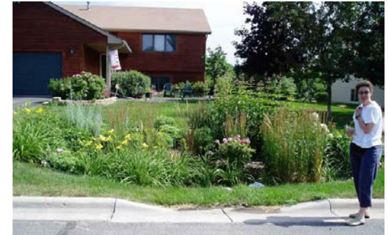
Rain gardens on individual lots provide opportunities for infiltration, but must be carefully maintained.
