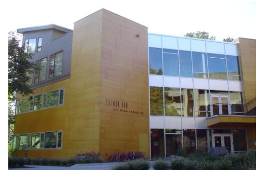
Mixed-use building includes office spaces and residential units on half of the upper level
