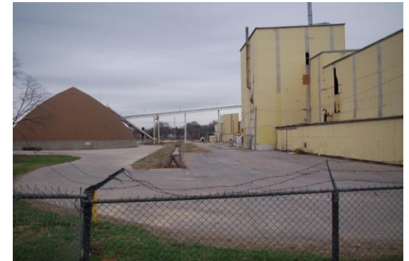
Exterior of the former Royster-Clark Fertilizer Plant, showing the main granulation building, one of two storage domes, and associated infrastructure
