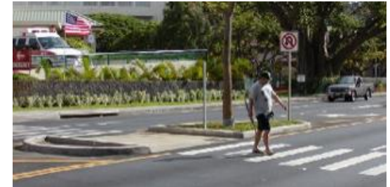
Pedestrian refuge island with crosswalk
