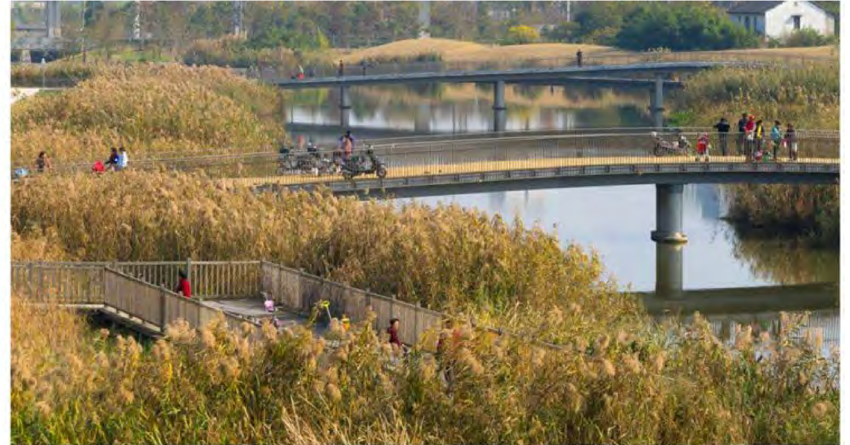
Wetland, Fish Habitat and Boardwalk
