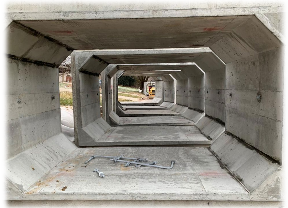
Photo of a box culvert (square stormwater pipe)
