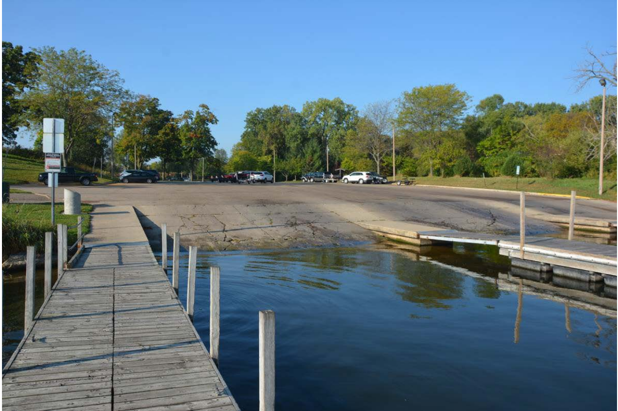
Existing boat landing facilities. View to southwest.
