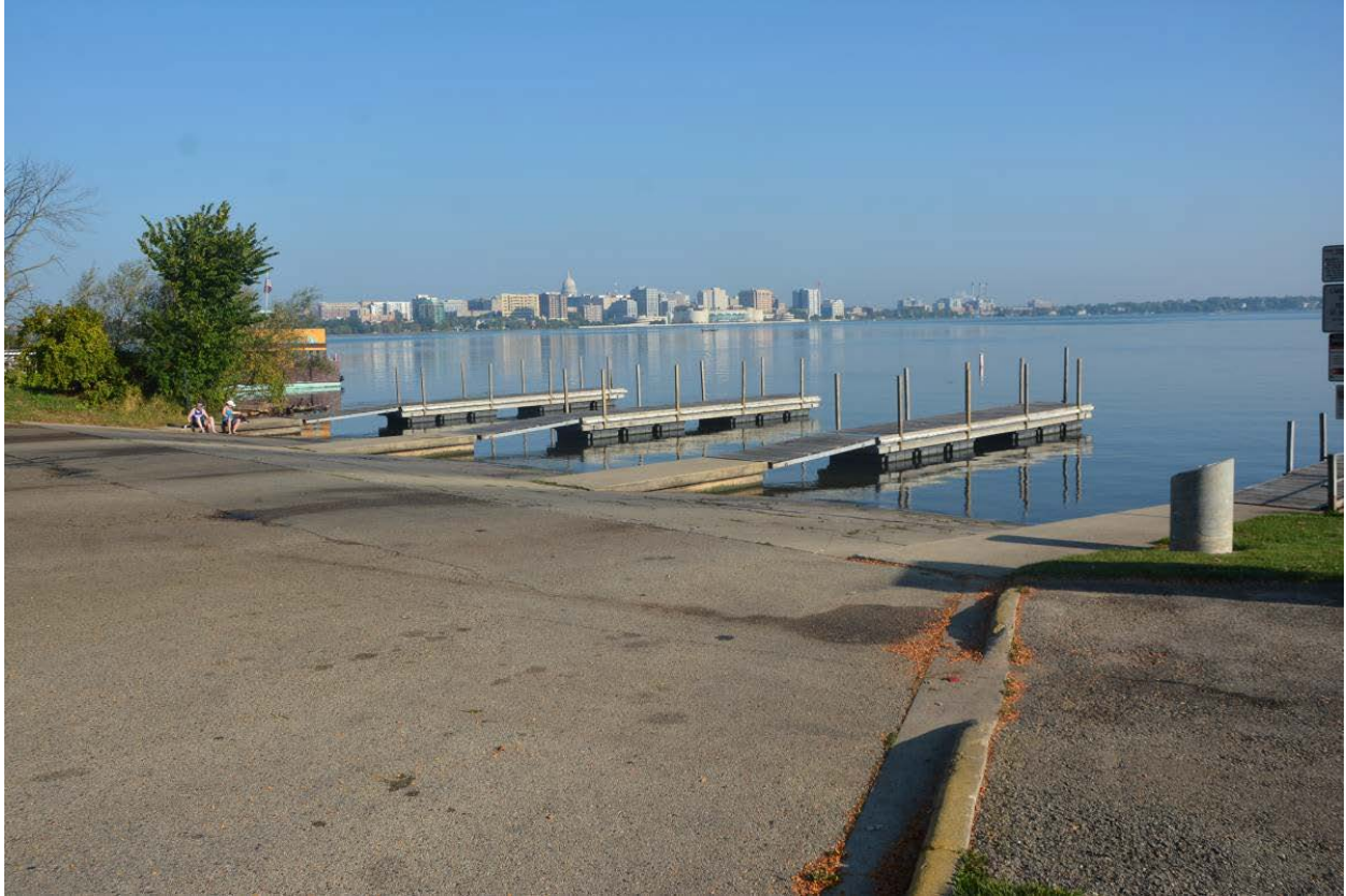
Existing boat landing facilities. View to north.
