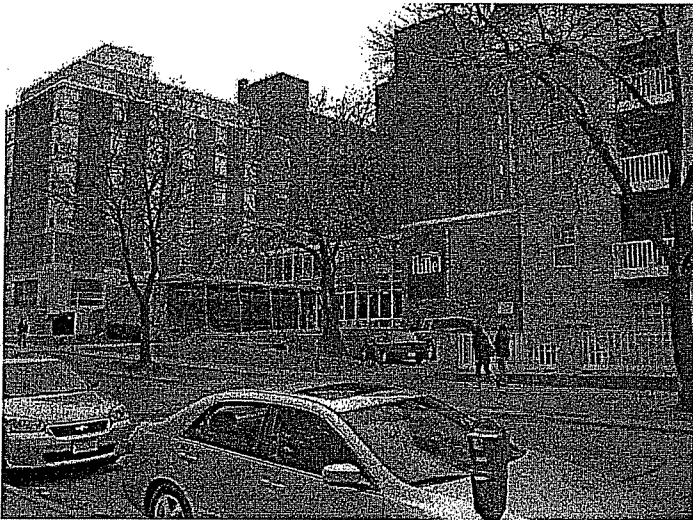
Figure 1. View From Langdon Looking Southeast
