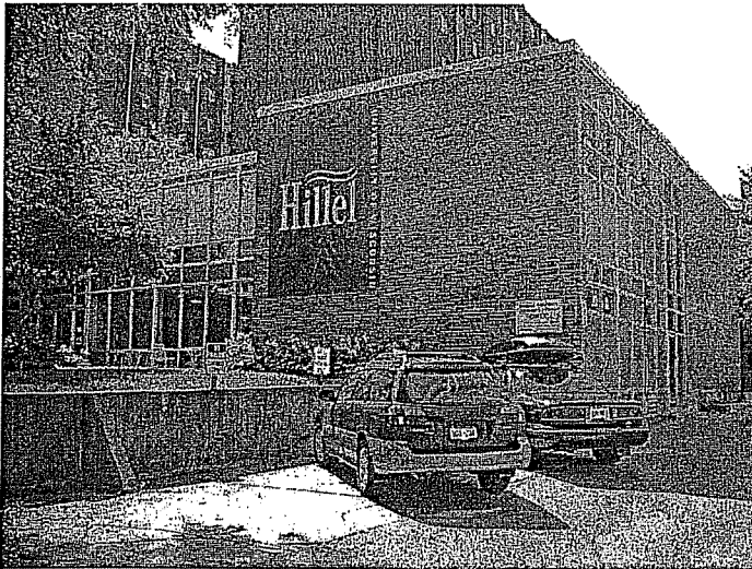
Figure 4. View From Alley Looking Towards The North Elevation
