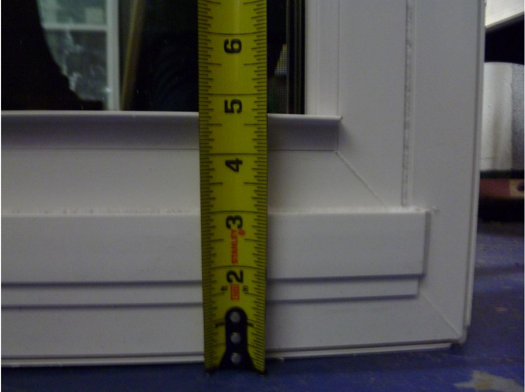
(Picture #6) 6000 SERIES DOUBLE HUNG BOTTOM PROFILE:
