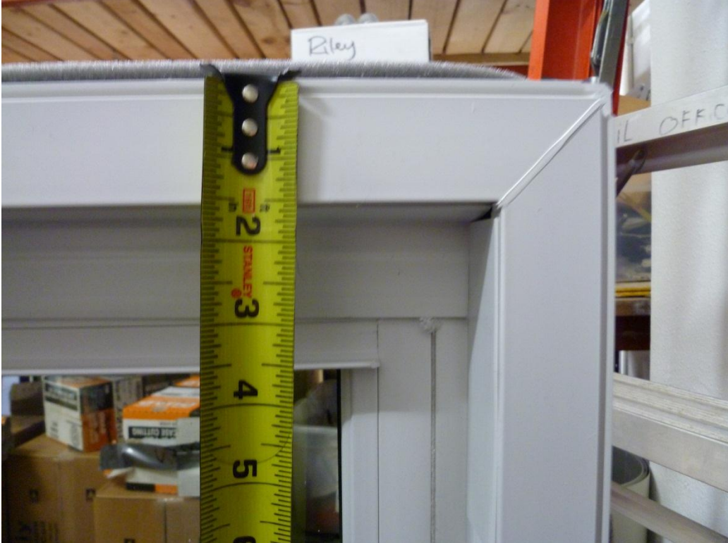
(Picture #5) 6000 SERIES DOUBLE HUNG TOP PROFILE:
