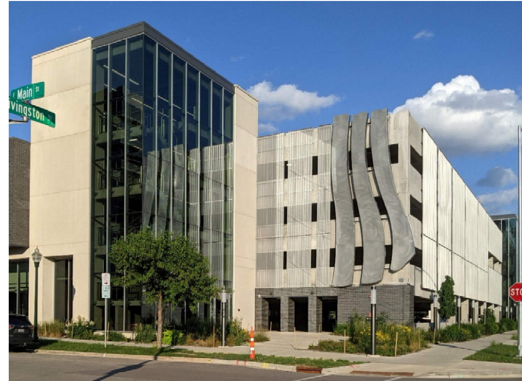
Exterior of City of Madison's Livingston Street Parking Structure showing the exterior materials: Brick, Perforated Metal, Concrete, Aluminum Curtainwall and glass, as well as the incorporation of public art.
