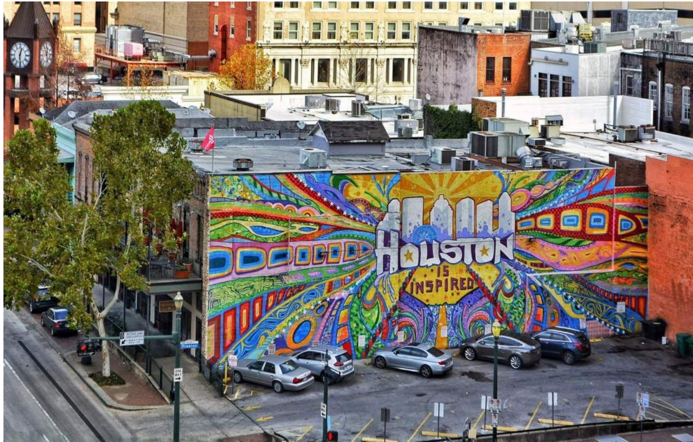
Example of a large public art mural on the side of a building that reflects the community
