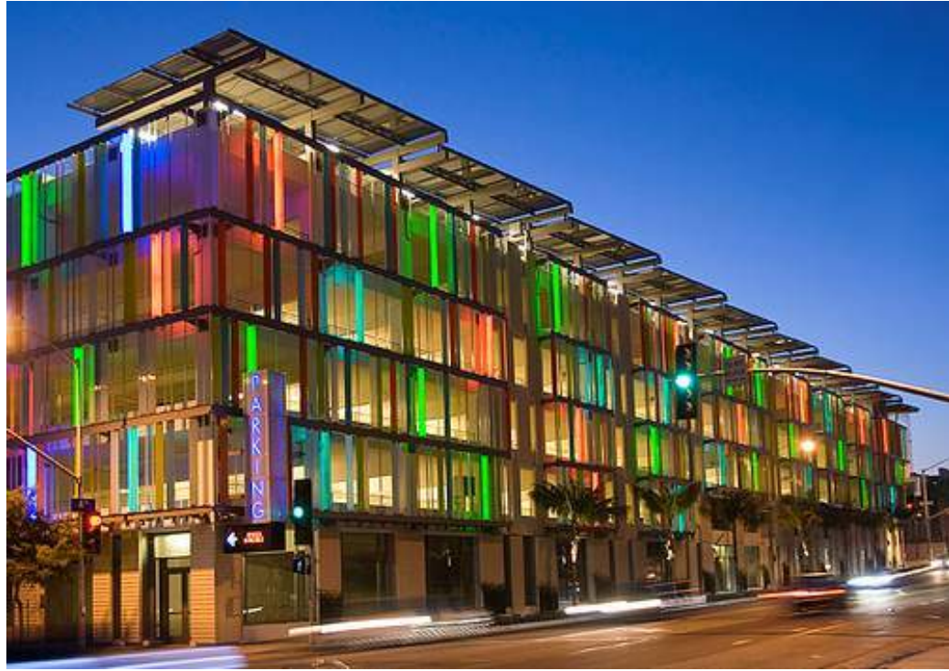
Santa Monica, CA: Colored glass panels and solar panels shading the roof
