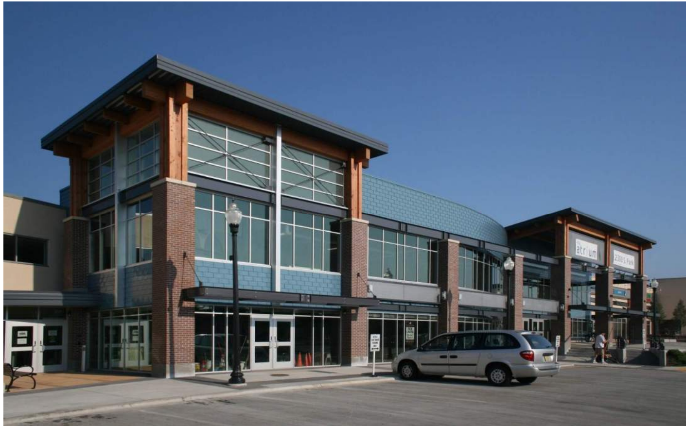
Exterior of existing Village on Park Main Building showing material palette
