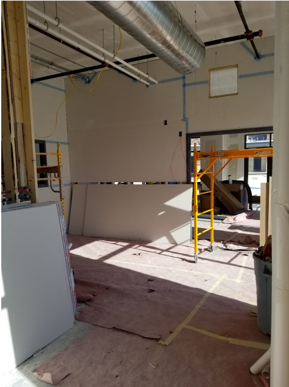
Brewspace plumbing and electrical completed, putting up FRP/drywall
