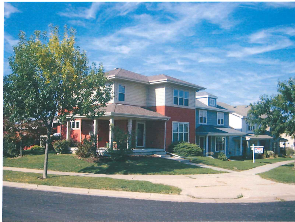
9—NORTH STAR DRIVE LOOKING NORTHWEST
