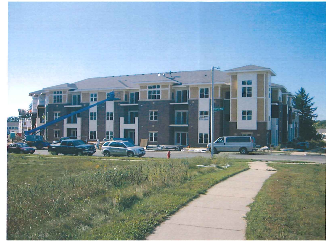
10—HERCULES TRAIL LOOKING NORTHWEST
