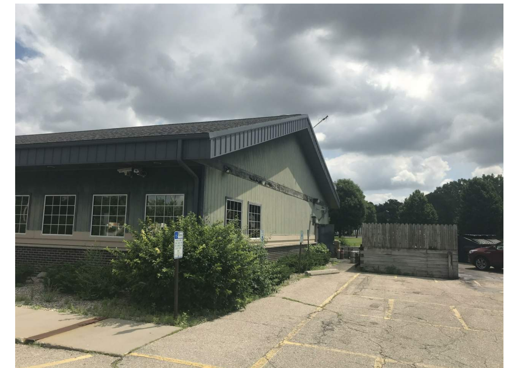
Existing Building South End - Looking to NE
