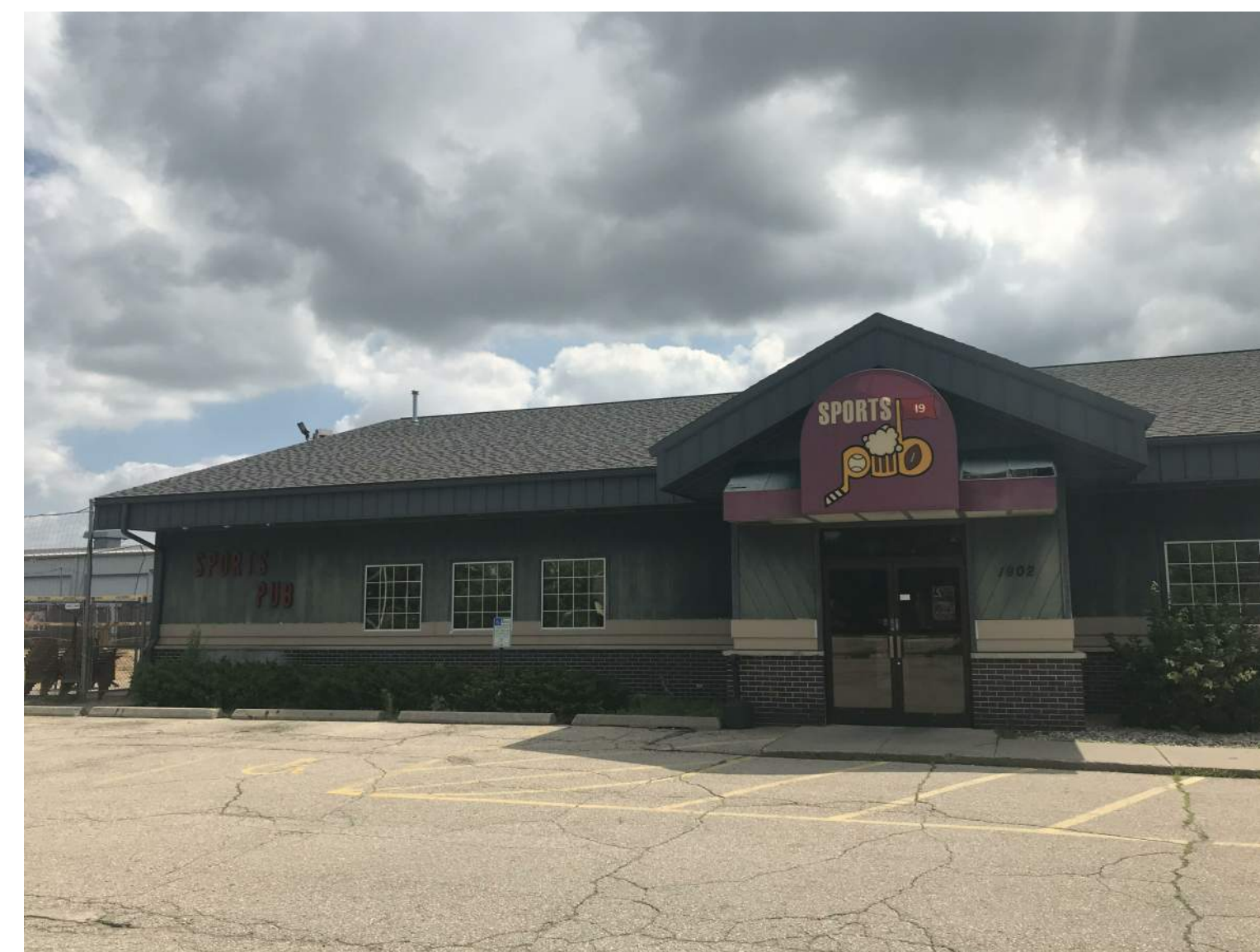
Existing Building West Entry - Looking to NE
