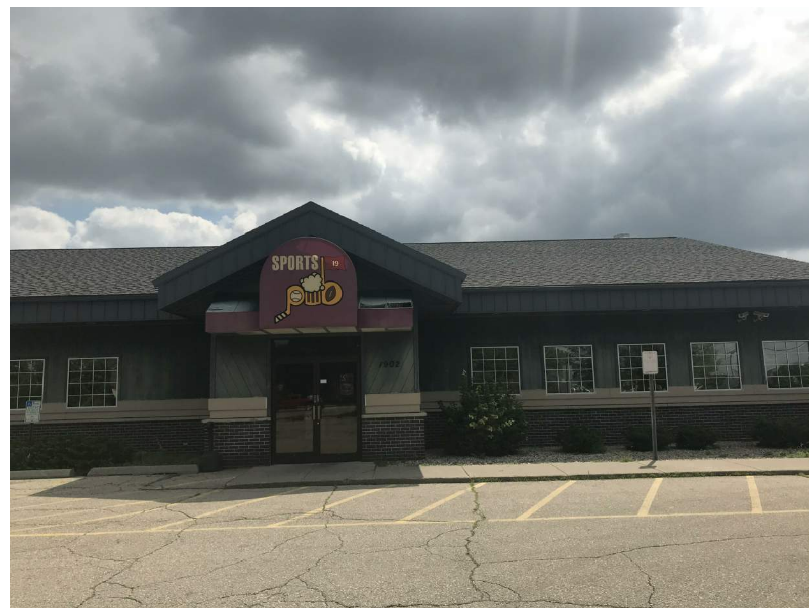
Existing Building West Entry - Looking to E
