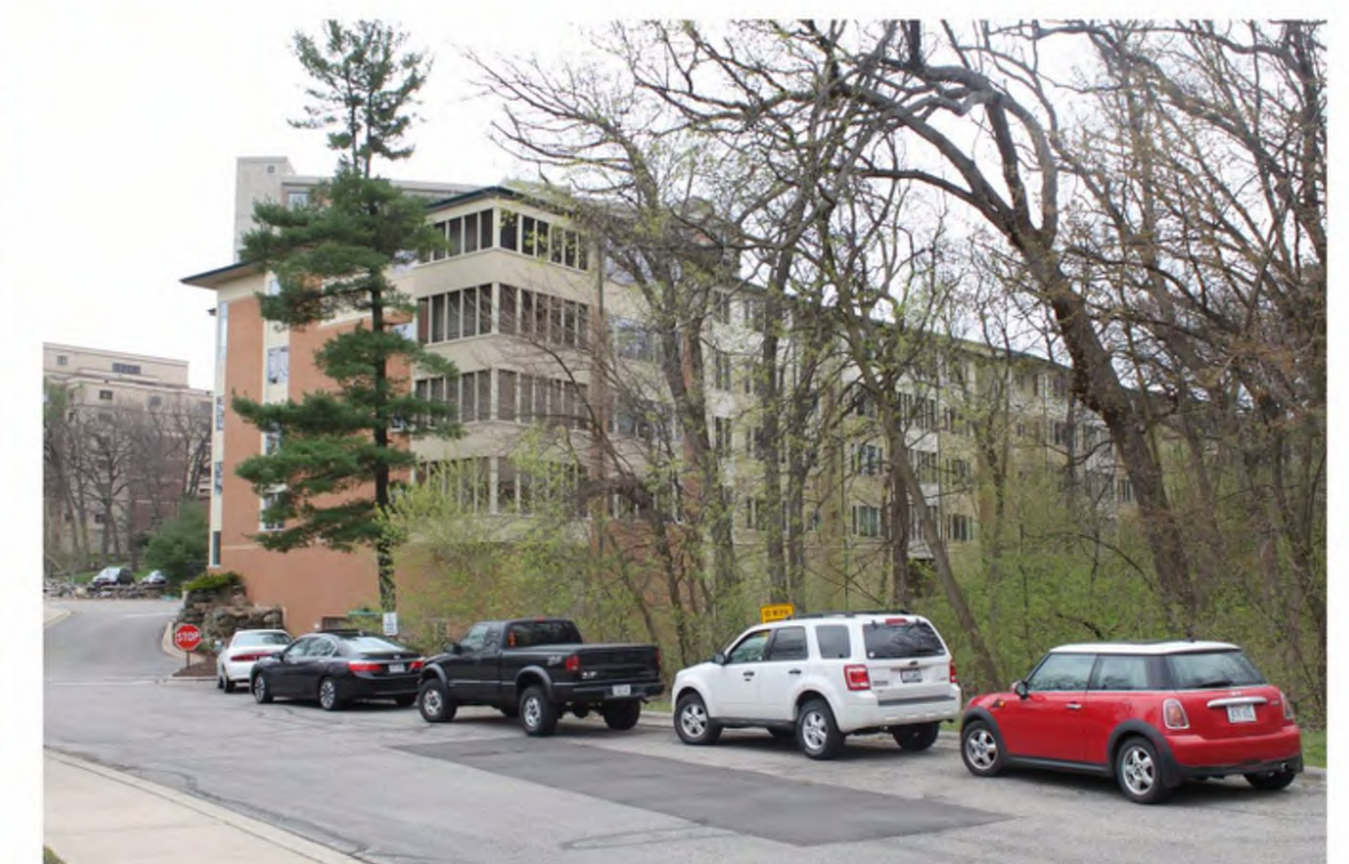
PHOTOS OF EXISTING SITE
