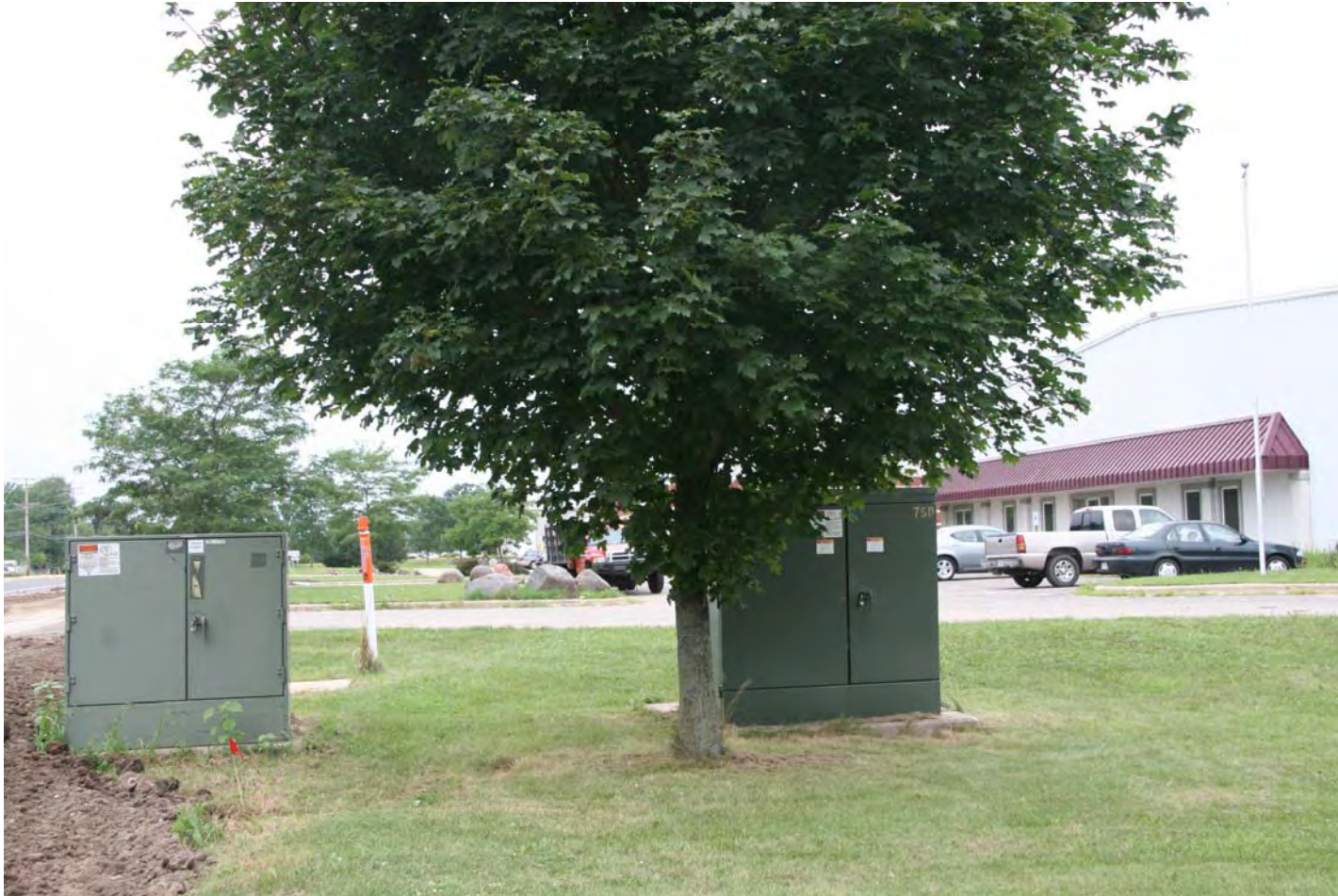
View to West of property
