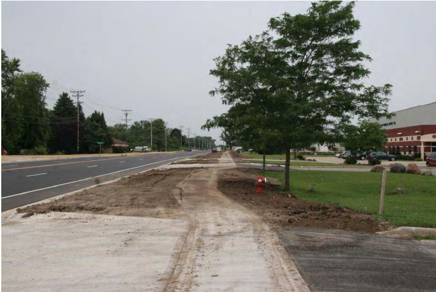
View to West of property
