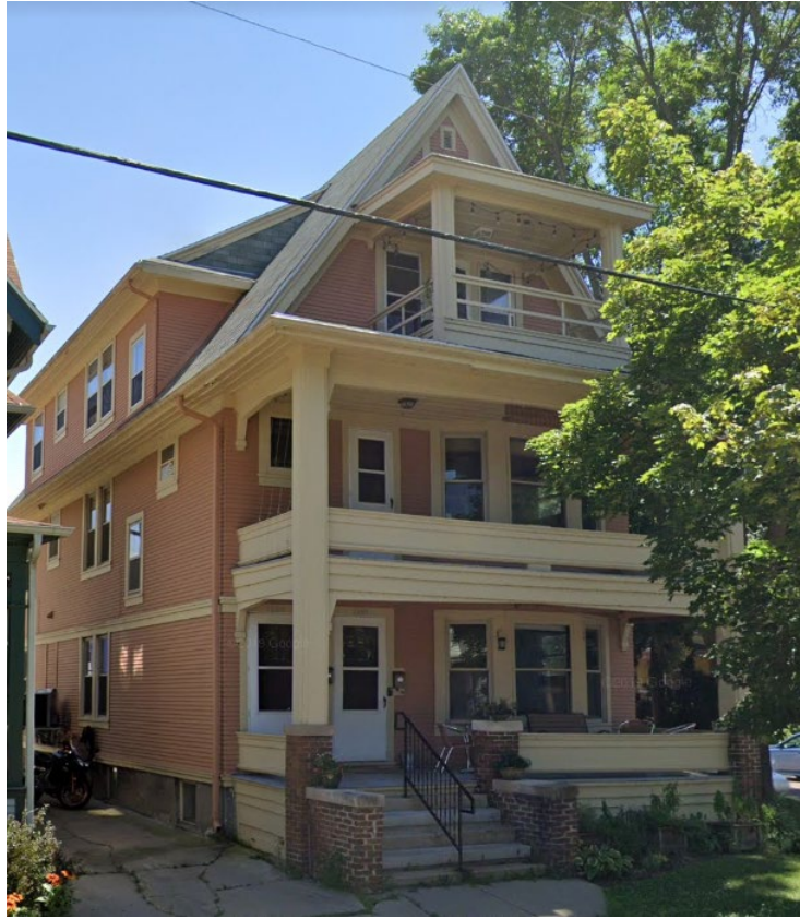
1201-1203 Jenifer Street (shed dormers on both sides)
