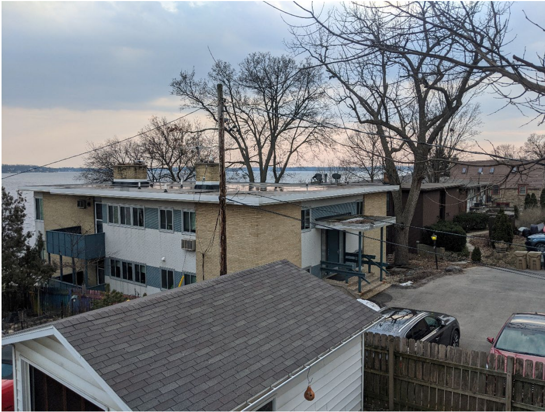
View of 1211 and 1219 Rutledge Street from rear of subject property
