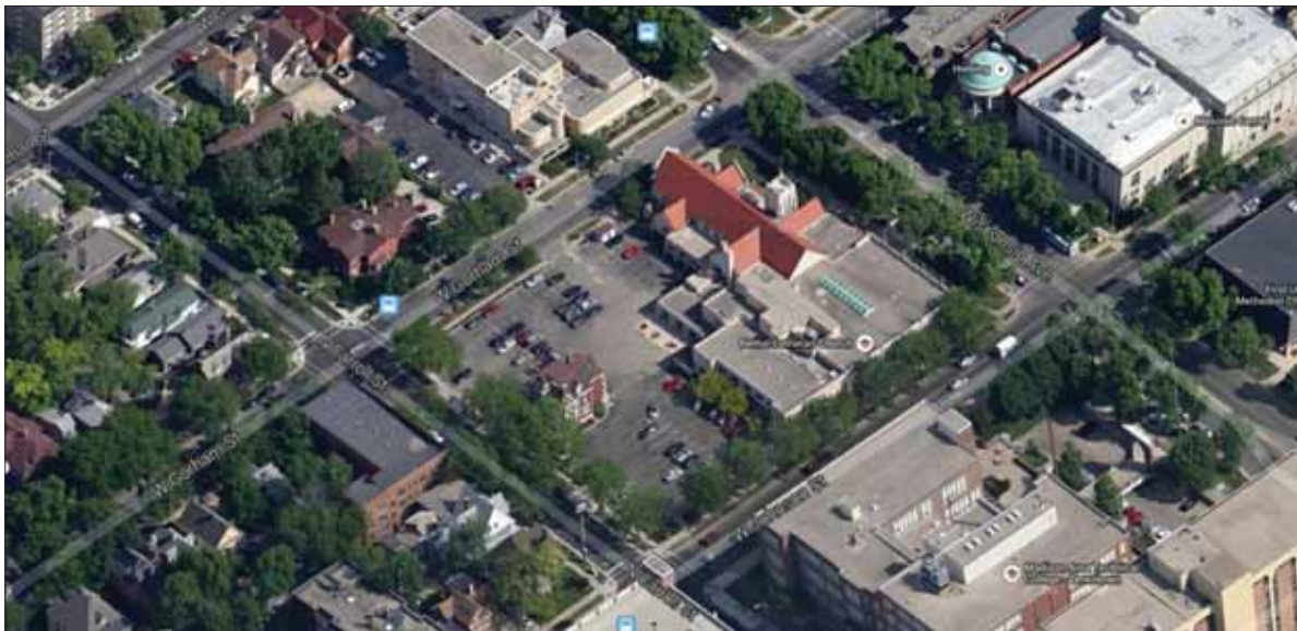
2 A100 AERIAL VIEW FROM SOUTH
