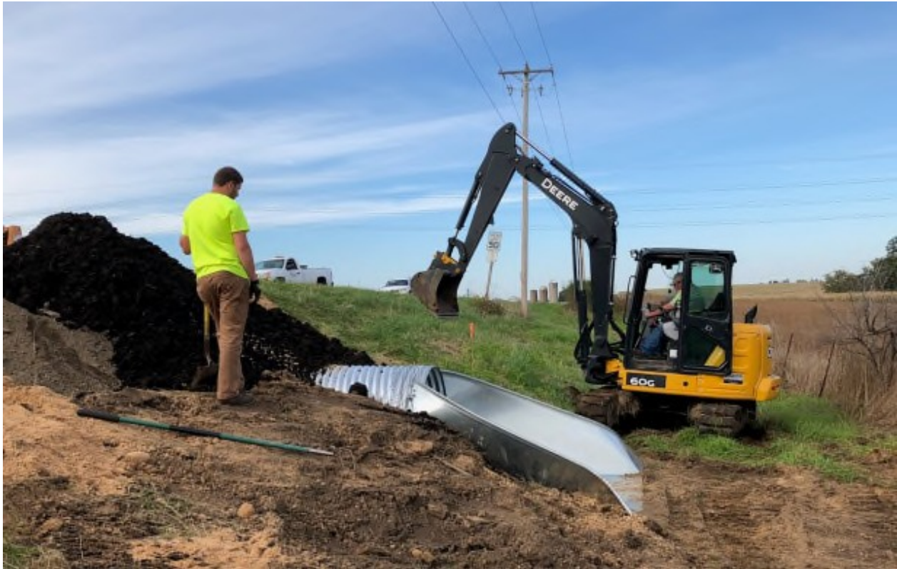
Figure 3-2. Culvert Replacement under Fitchrona Road
