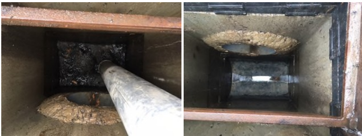
Figures 7-3 and 7-4. Sump during and after Sediment Removal
