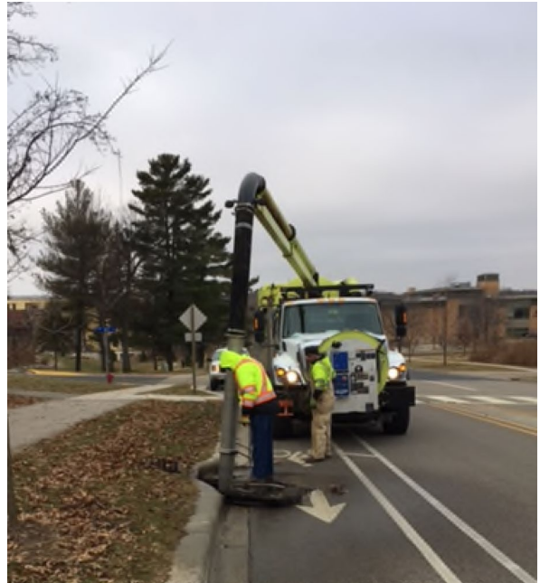
Figure 7-2. Public Works crews remove sediment from Sumps on Lacy Road
