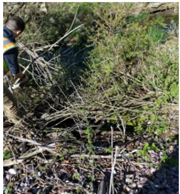
Figure 3-5: Public Works staff clear tree Branches blocking an Outfall
