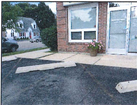
Front façade lower left detail
