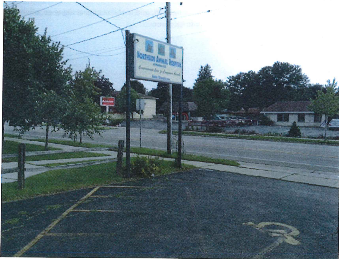
Parking lot facing west. Sign posts to be painted; caps added to top of posts.
