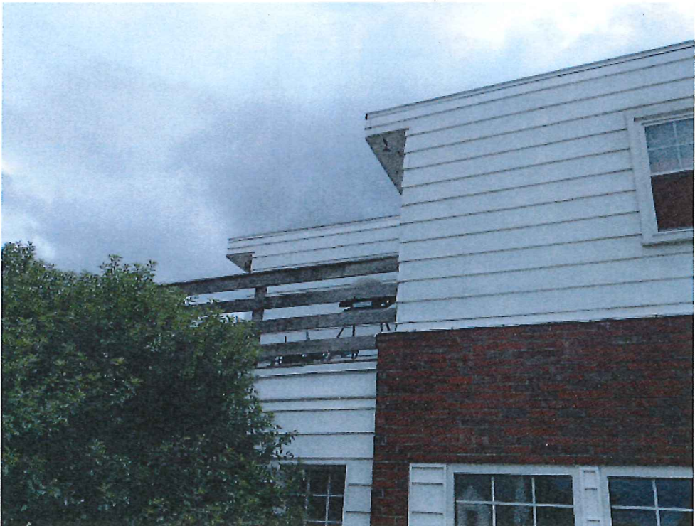
Vahlen façade-east detail.
