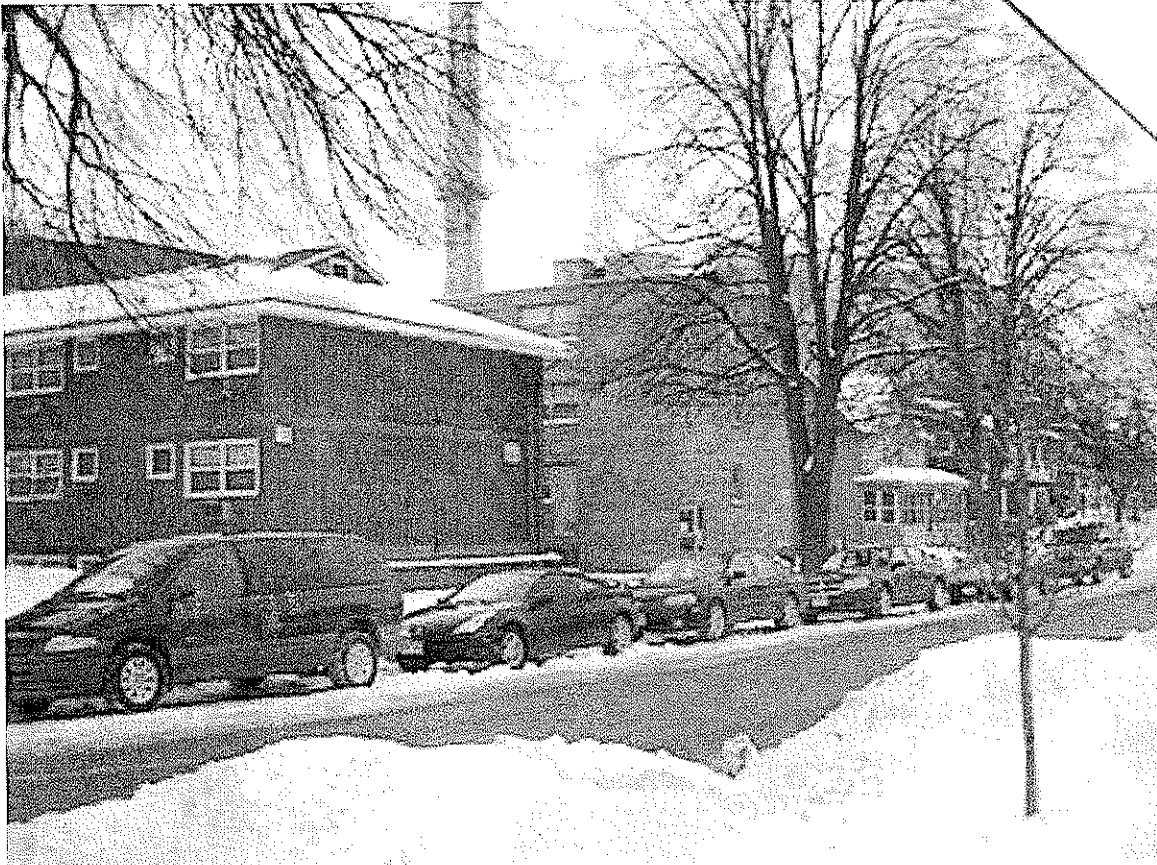
View of subject properties to northeast from Spring Street
