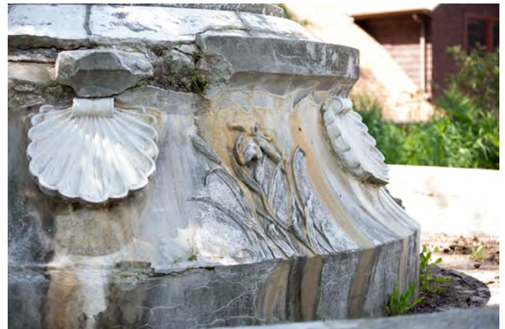
Figure 22: Overall condition of stone base - the damage is excessive and beyond repair
