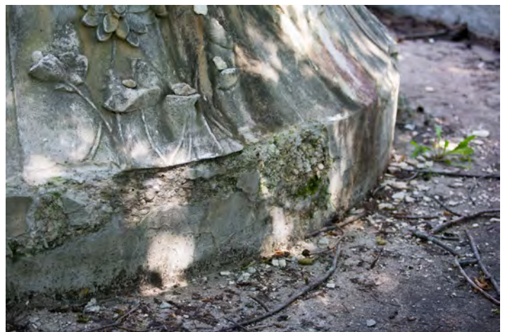
Figure 31: Stone to concrete transition
