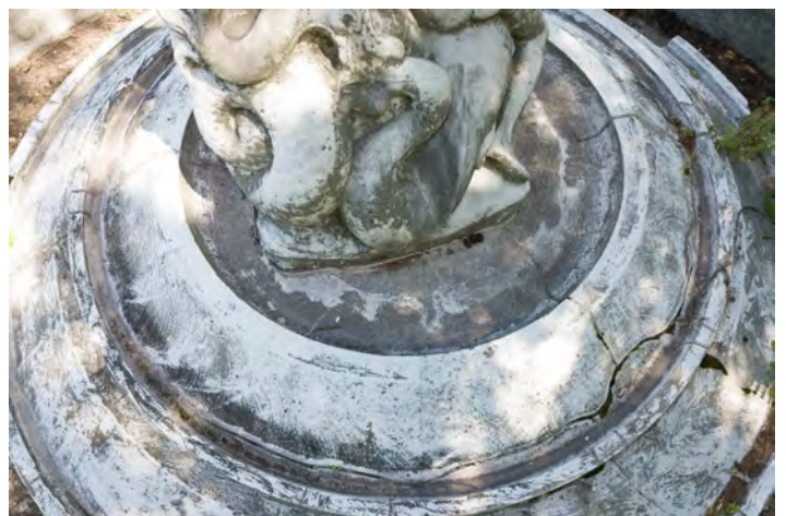
Figure 7: Upper view of pedestal and base - note damage to pedestal has been repaired and appears to have stabilized
