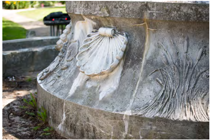
Figure 35: View of relief at foundation base
