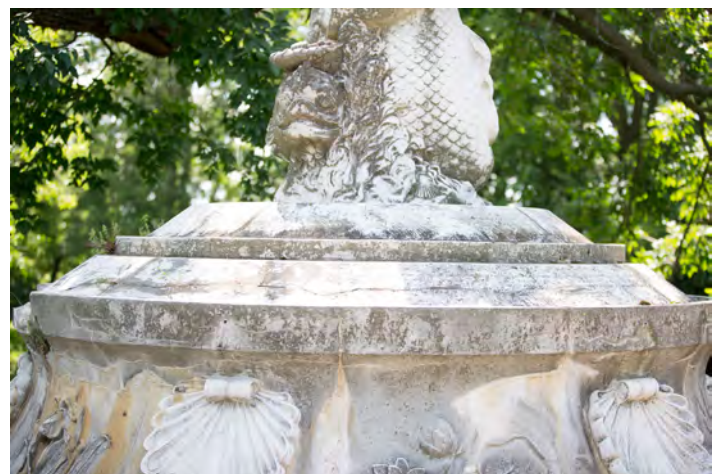
Figure 19: Relatively intact base/pedestal transition
