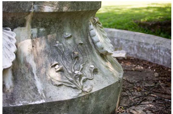
Figure 33: View of relief at fountain base
