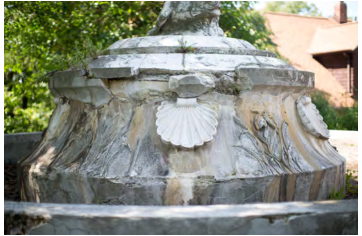
Figure 44: Overall view of base
