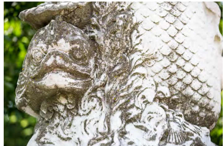
Figure 54: View of dolphin in 2017
