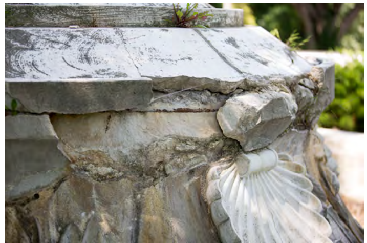
Figure 42: View of damage at tension ring
