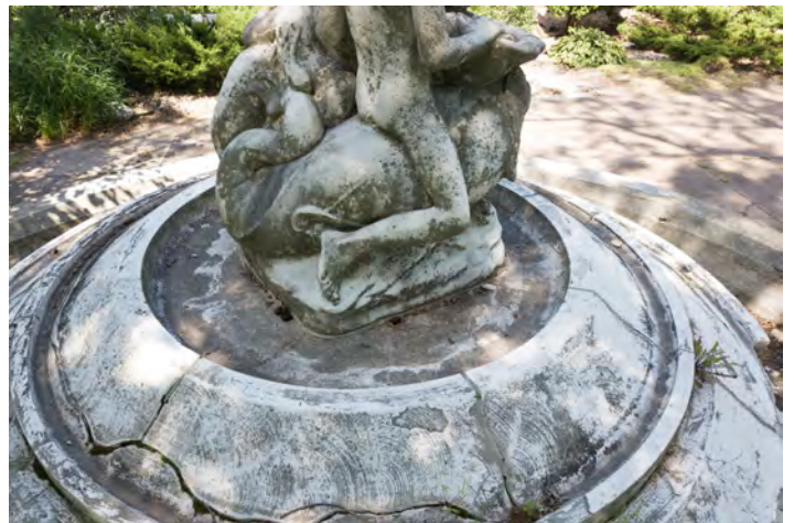
Figure 6: View of marble figures and upper view of pedestal and base - note damage to pedestal has been repaired and appears to have stabilized
