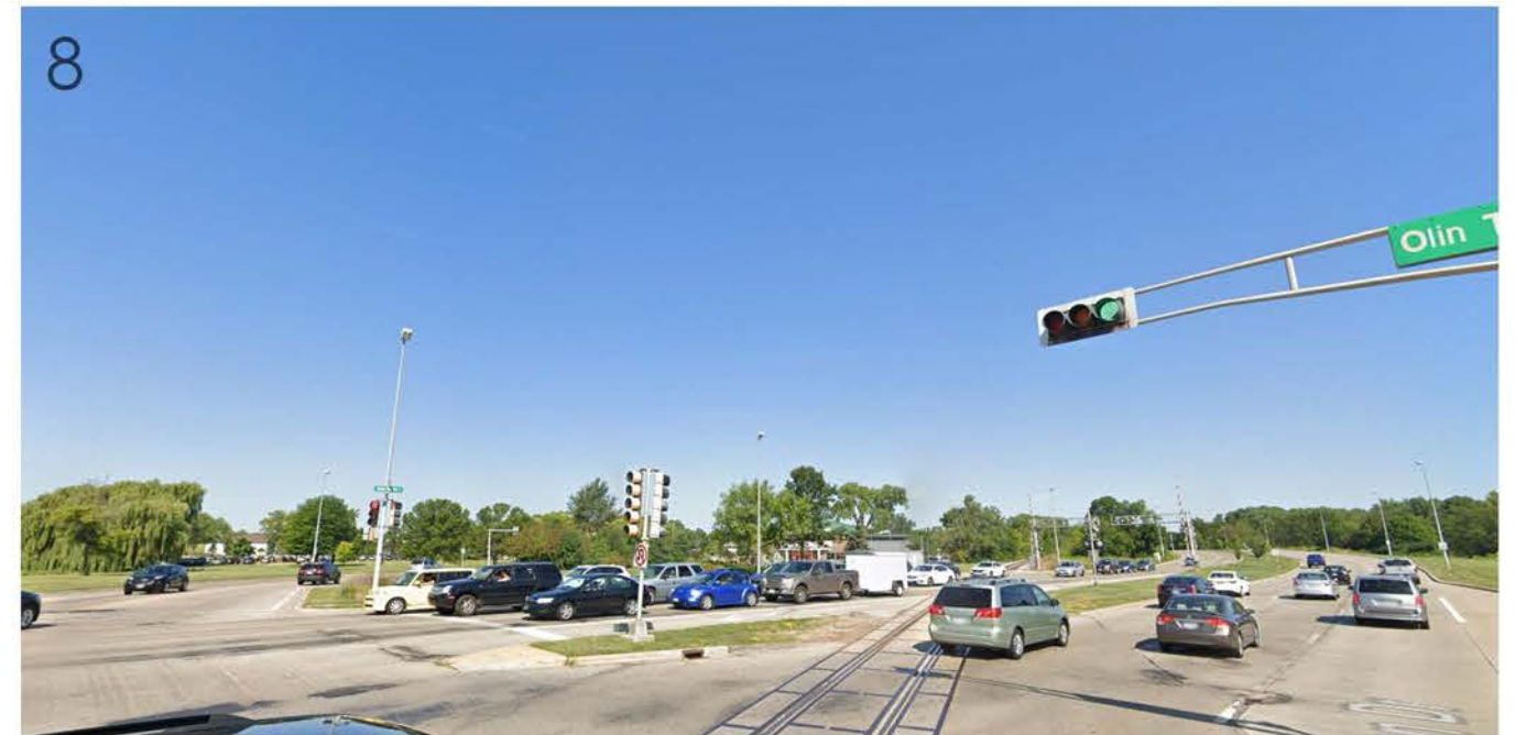
8: OLIN-TURNVILLE CT - FACING WEST
