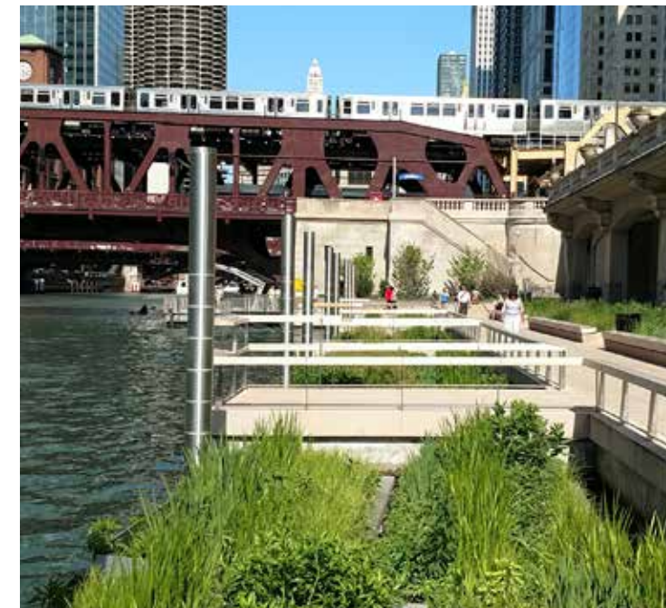
Collins Engineering Inc. Riverwalk Extension, Chicago IL
