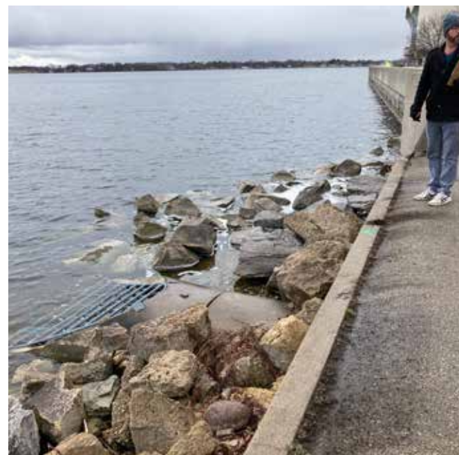
Image from team site visit, City of Madison WI
