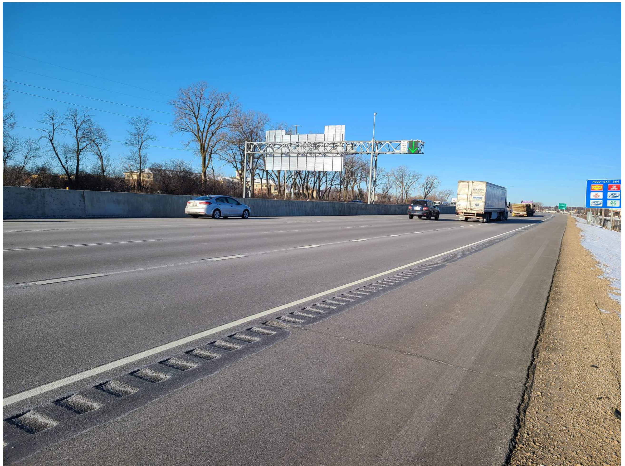
CONCRETE MEDIAN BLOCKS VIEW FROM EASTBOUND BELTLINE
