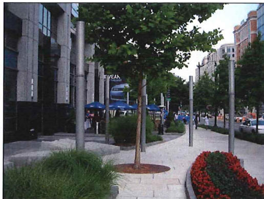
Soil areas under suspended pavement and root paths connect trees to landscape areas on K St., NW.
