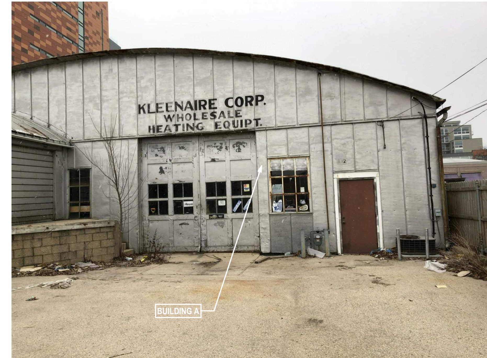
EXISTING PHOTO- EAST ELEVATION-BUILDING A
