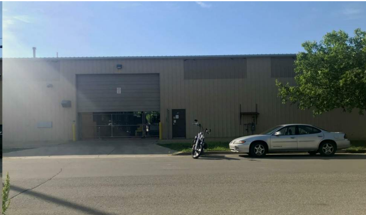
Mechanical Shop and Storage
