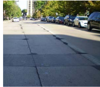
Carroll looking NW (asphalt patching)
