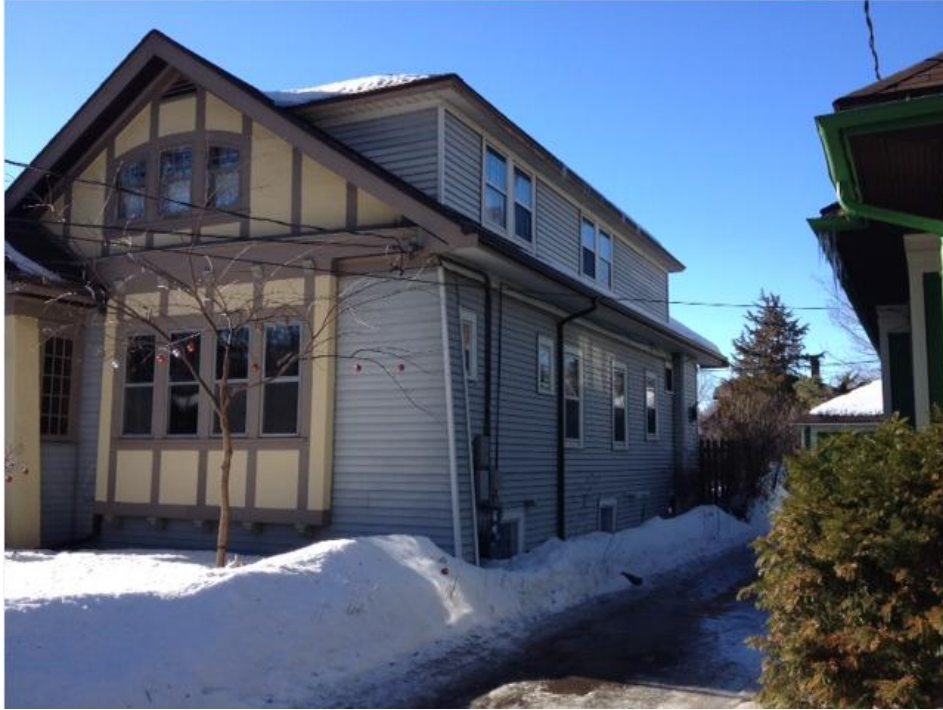
15. Right Side of Home – windows, siding and soffit
