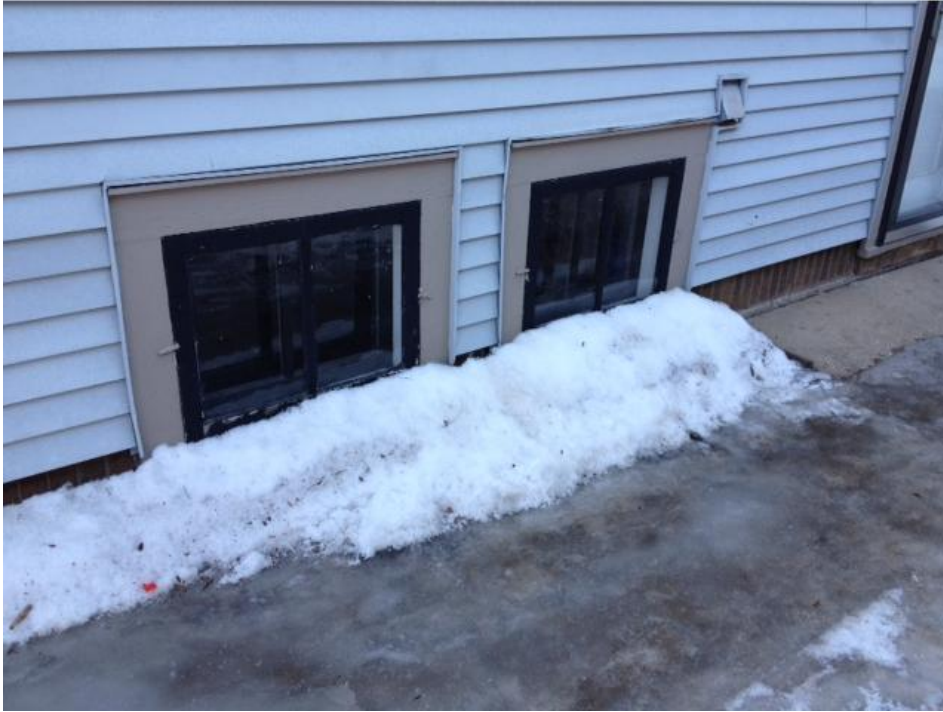
11. Left Side Basement Windows - replace with matching Andersen windows
