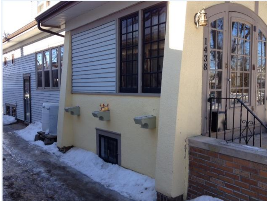
8. 1 st Floor Side Vestibule Windows - replace with matching Renewal by Andersen
