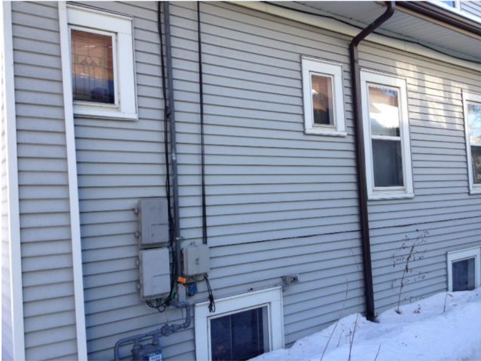
16. 1 st Floor Right Side Windows - replace with matching Renewal by Andersen
