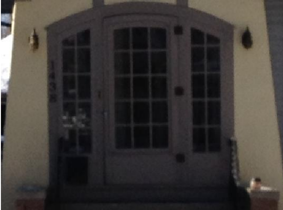
5. Front door and windows – maintain existing; no changes at this time
