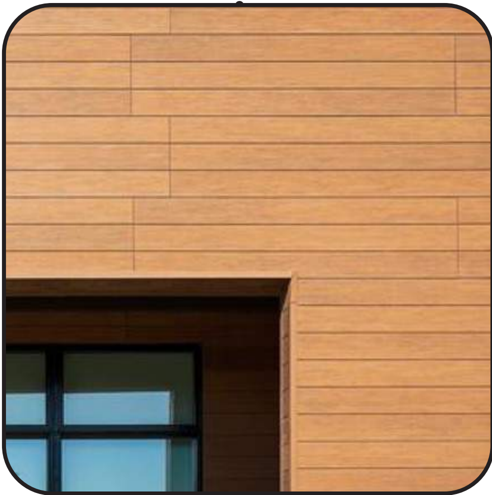
FIBER-CEMENT SIDING - ACCENT MATERIAL
