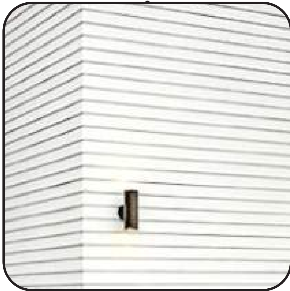
FIBER-CEMENT LAP SIDING
