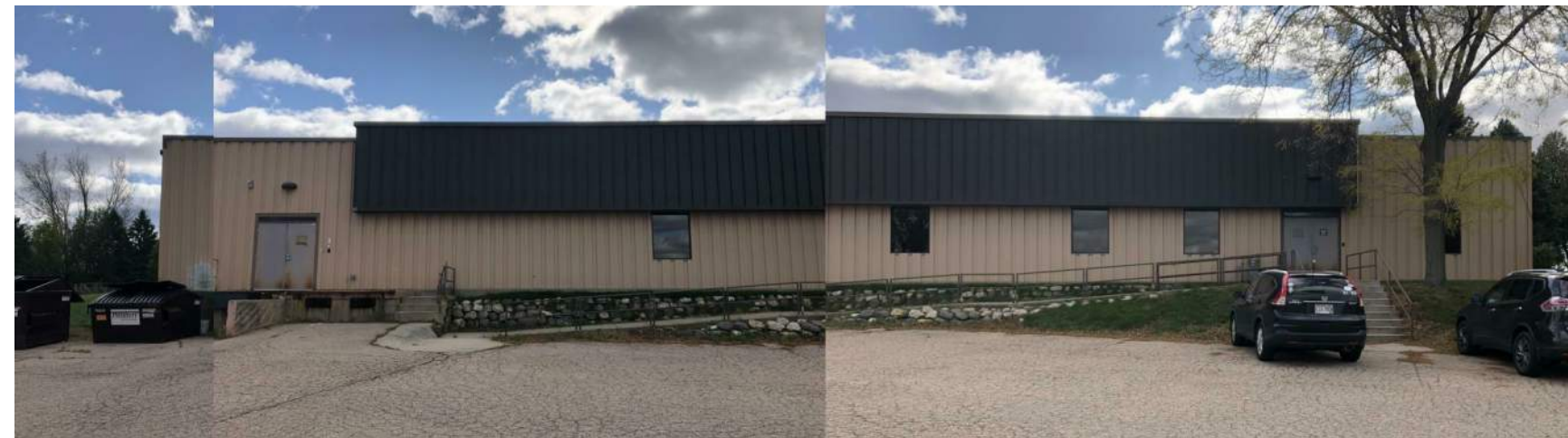
NORTH ELEVATION - EXISTING PHOTOS
