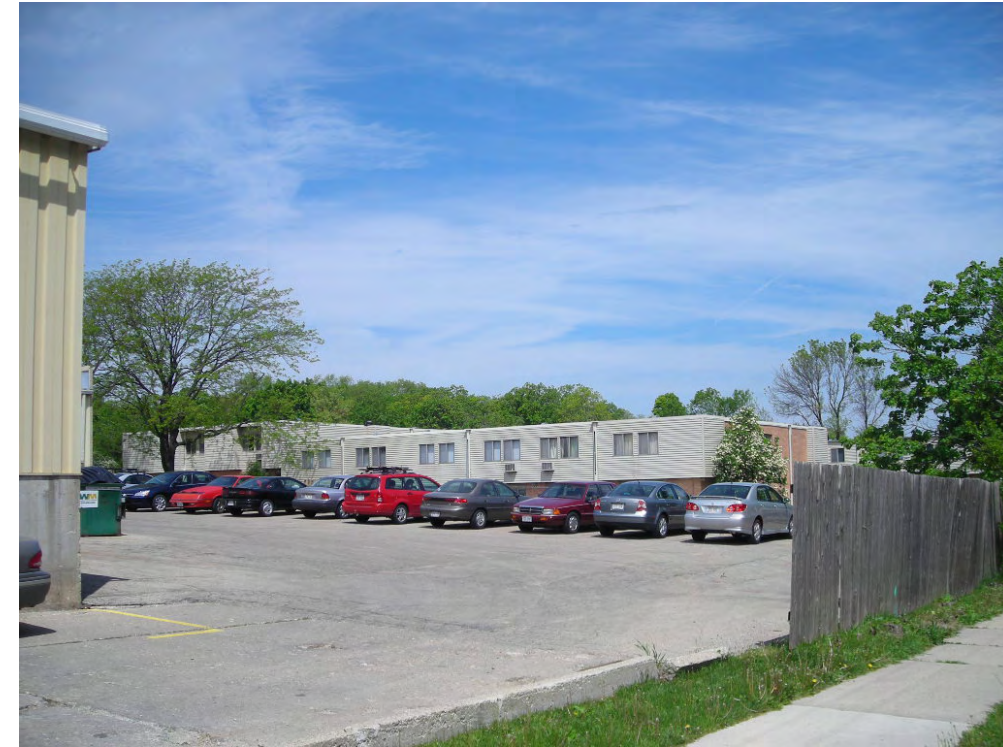
View North at Existing Apartments
