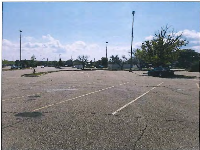
IMAGE 4: FROM SITE FACING WEST TOWARD ASSOCIATED BANK LOT
