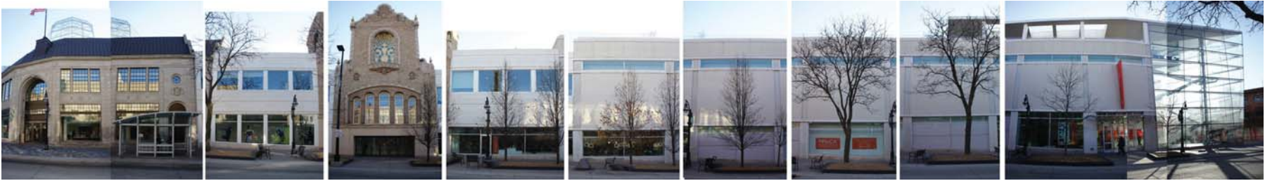
200 Block of State Street (South)
